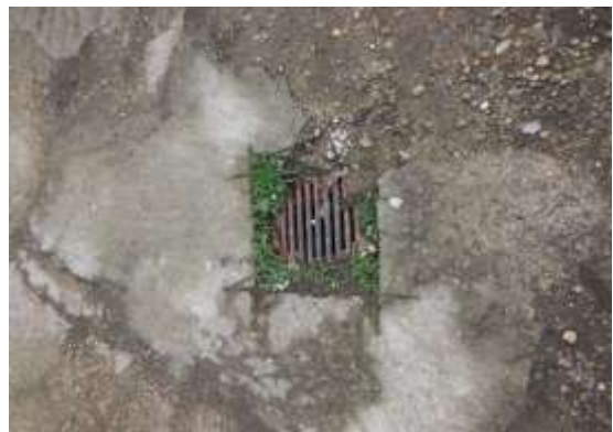
Figure 7 – Existing surface water gully
