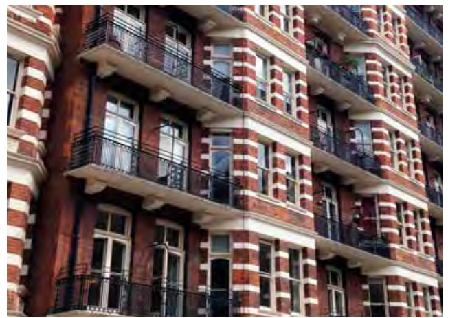
Wrapping balcony forms in mansion blocks
