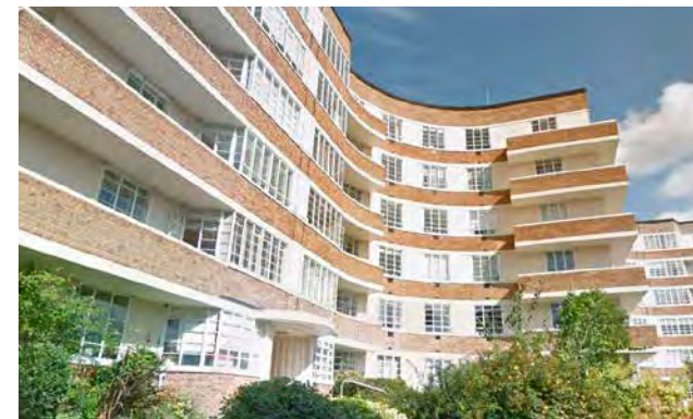
Elevational precedent 01 - Cholmeley Lodge
