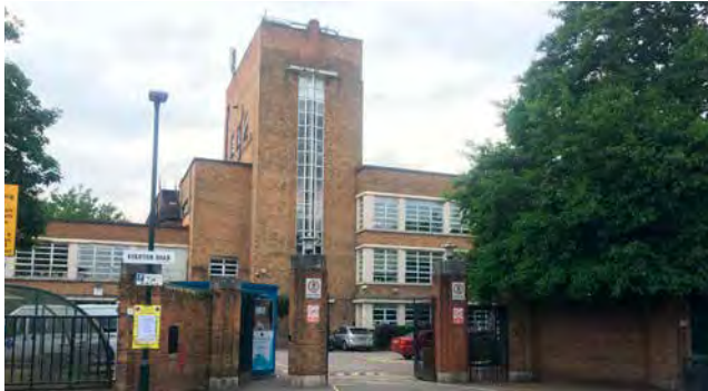
04 Existing Richmond upon Thames College building
