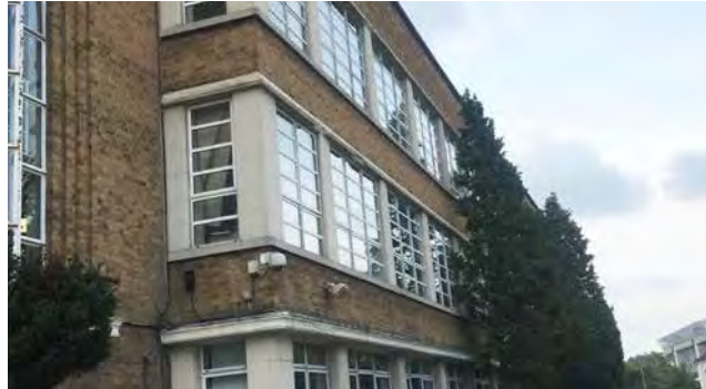
03 Existing Richmond upon Thames College building
