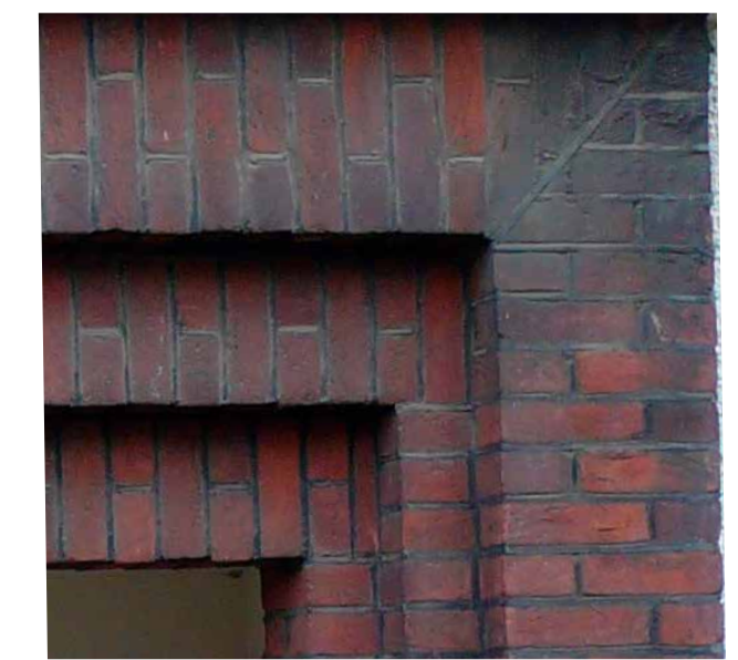
Brick work details and corbelling features. - Modern example above
