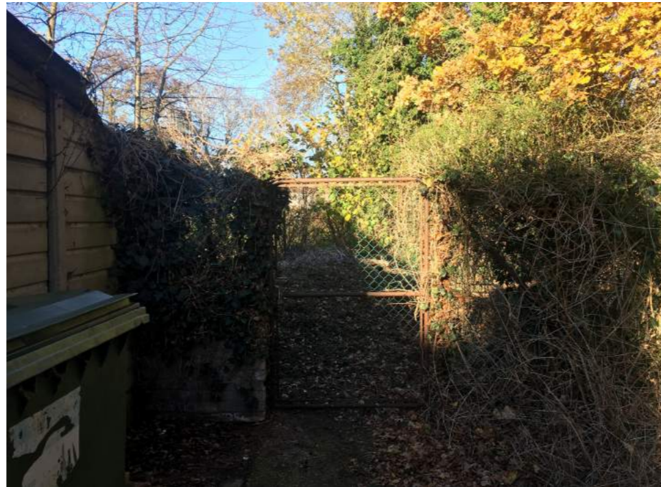
FIG. 28 VIEW 7 SIDE OF EXISTING GARAGE
