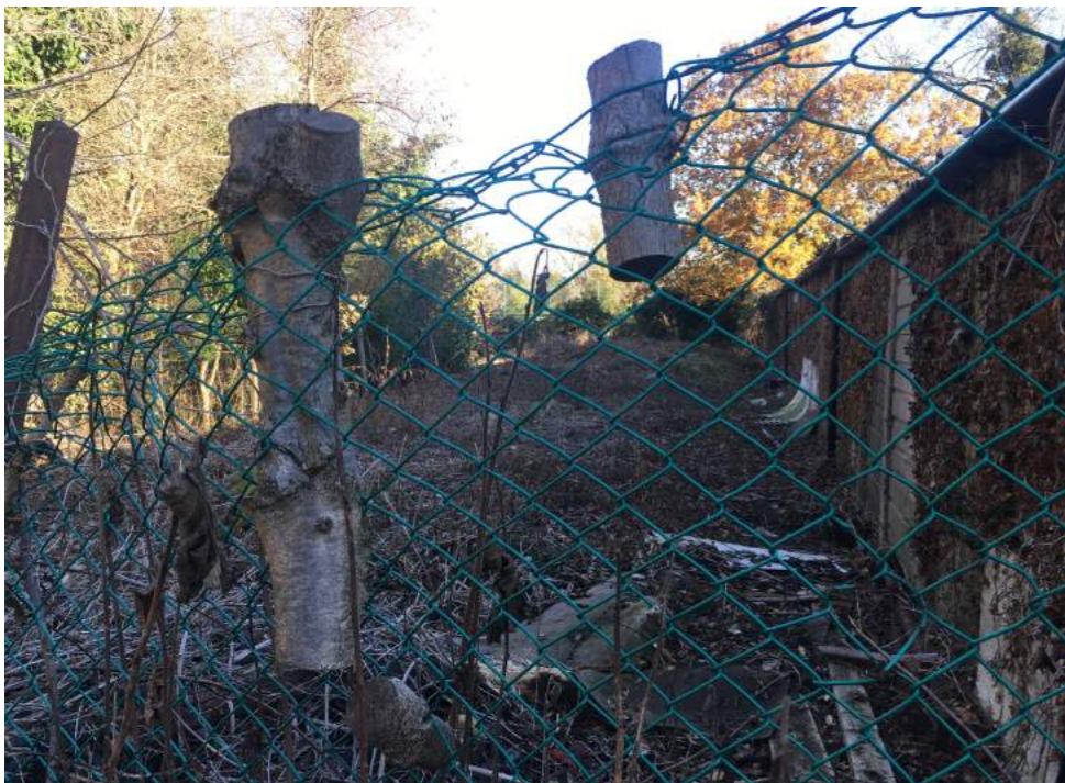
FIG. 30 VIEW 9 REAR OF EXISTING GARAGE WITH OVERGROWN VEGETATION AND DUMPED RUBBISH
