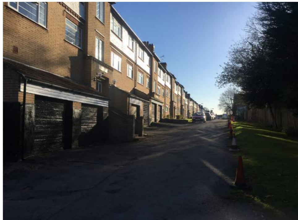
FIG. 31 VIEW 10 LOOKING SOUTH EAST TOWARDS NO.72-75 CHURCHVIEW ROAD
