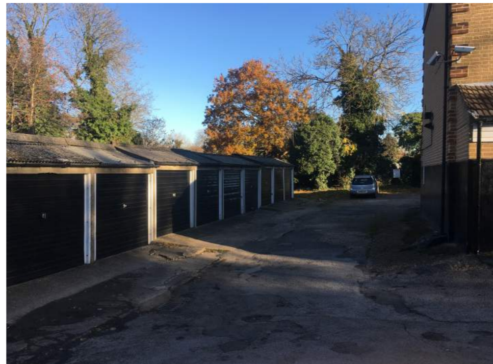
FIG. 15 VIEW 5 EXISTING GARAGE LOOKING NORTH EAST
