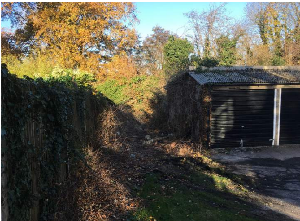
FIG. 14 VIEW 4 EXISTING GARAGE LOOKING NORTHWEST
