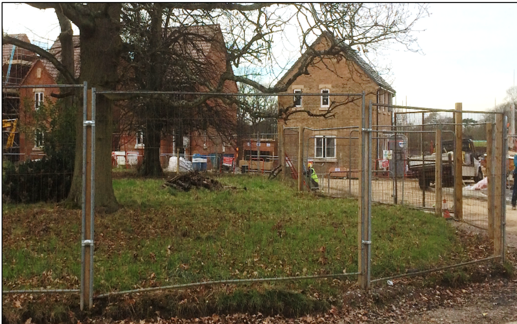
Weld-mesh panels on wooden posts
