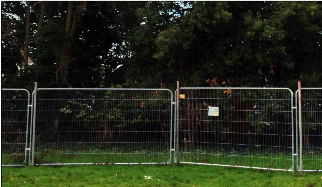
Weld-mesh panels on scaffold uprights
