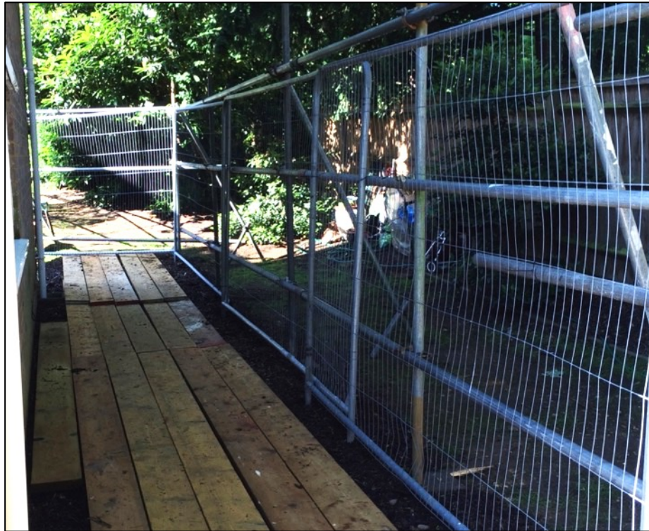
Scaffold board pedestrian ground protection
