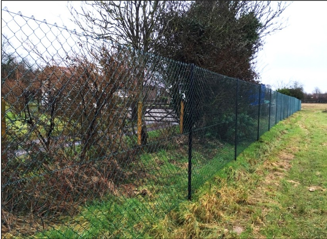
Chain-link on angle-iron uprights
