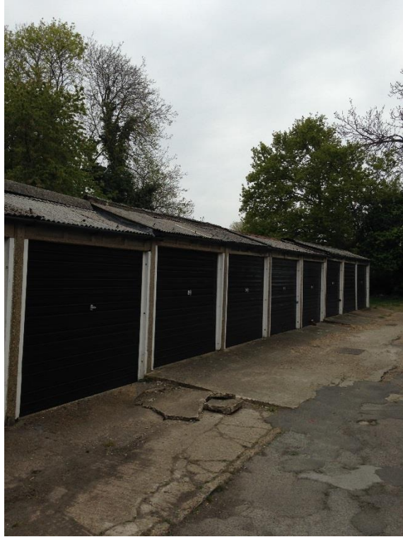
Photograph 1: View of garages, south east elevation.
