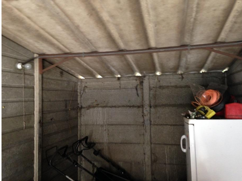
Photograph 3: View of garage interior.
