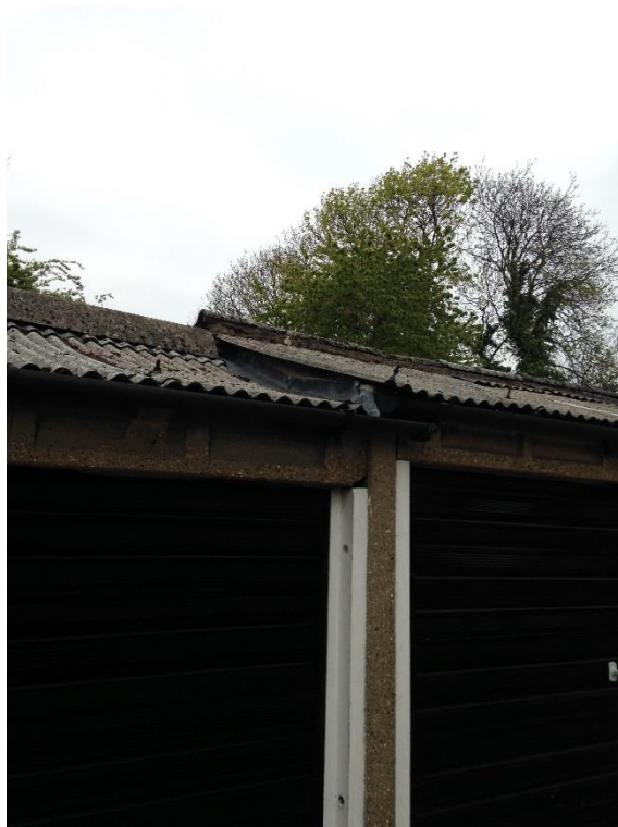
Photograph 2: View of garage roof.
