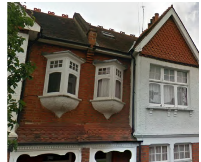
Angled Windows and Decorative Gable Treatment
