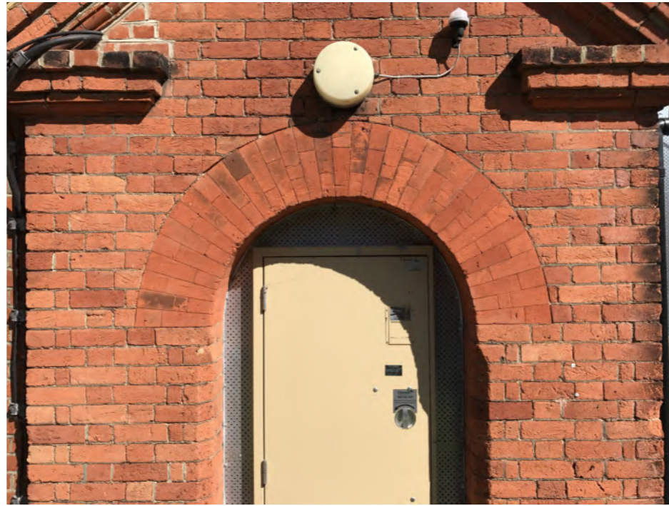
Gauged Brickwork, on site
