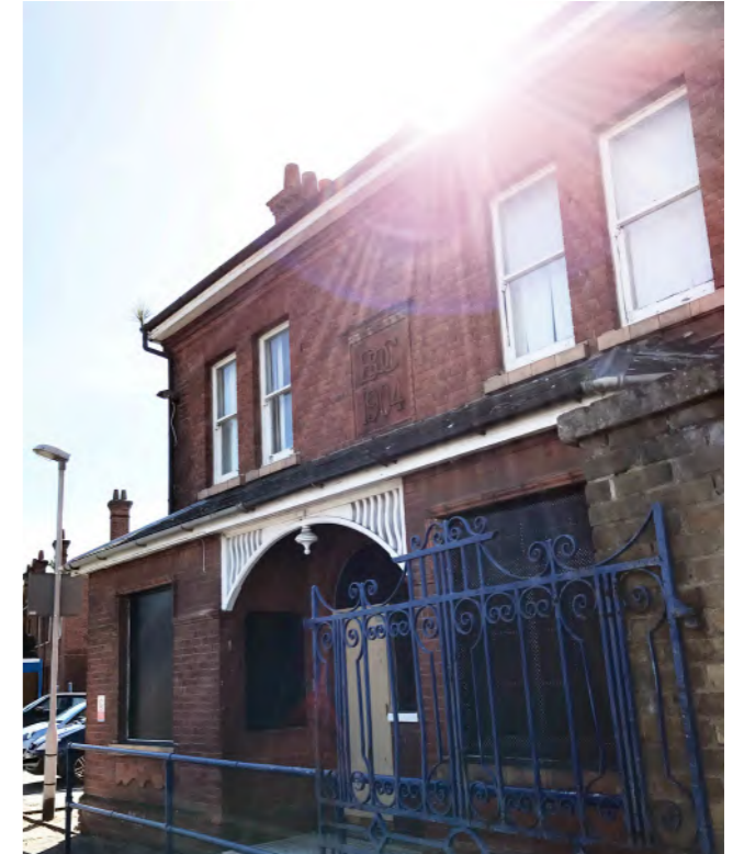
The Entrance Lodge [B]
