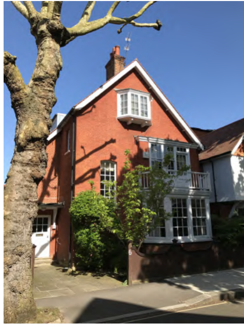
Angled Bay Windows, Bedford Park
