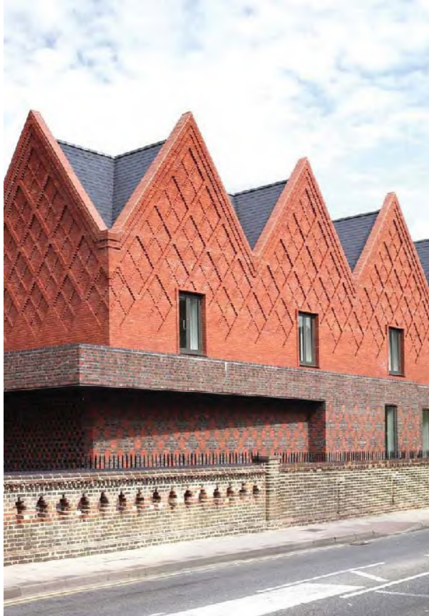
Example of contemporary detailing of vernacular form
