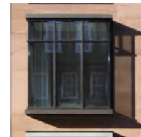
Metal work of lead / zinc to balustrades and window bays
