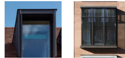
Metal work of lead / zinc to balustrades and window bays
