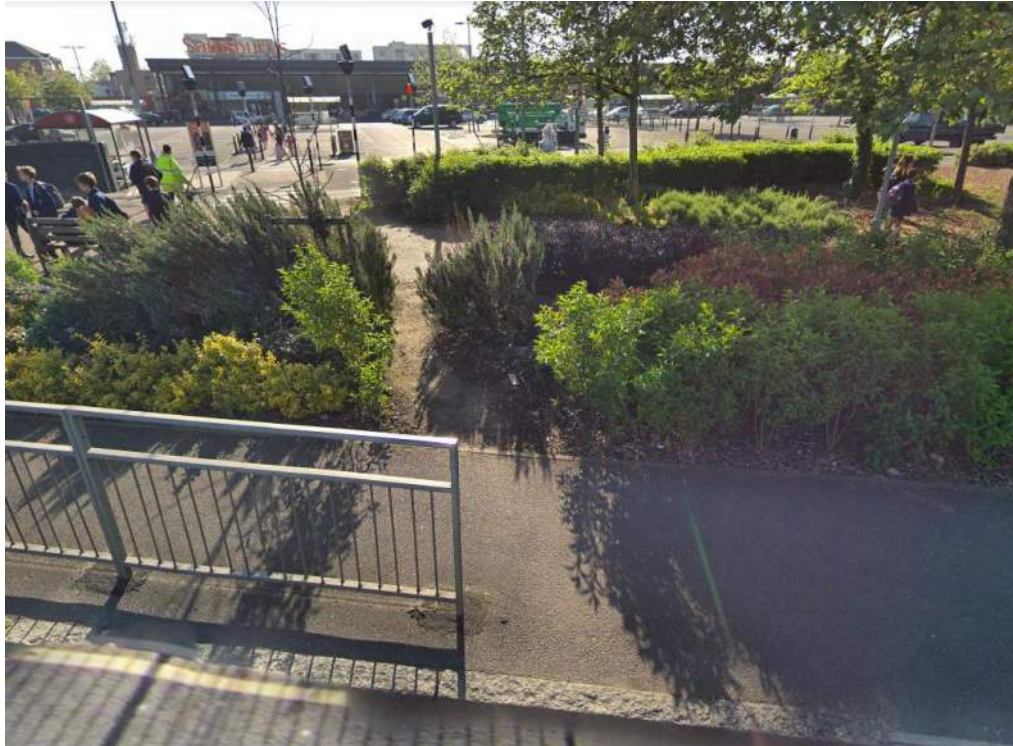
Figure 6 - Pedestrian worn path through Sainsbury's landscaping (©2019 Google)
