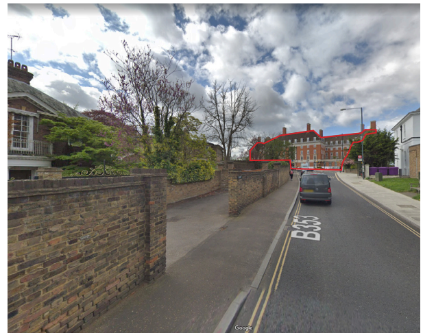
Royal Star and Garter Home - 8 storeys surrounded by 2 storeys. Stately scale reflects the building's prominence in its surroundings.
