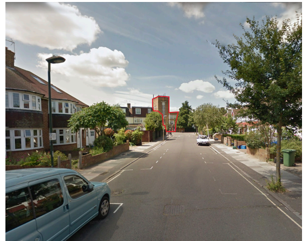
Richmond Upon Thames college - 5 storeys surrounded by 2 storeys. Taller element signifies the civic building use.
