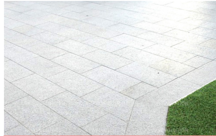
Granite paving with frame
