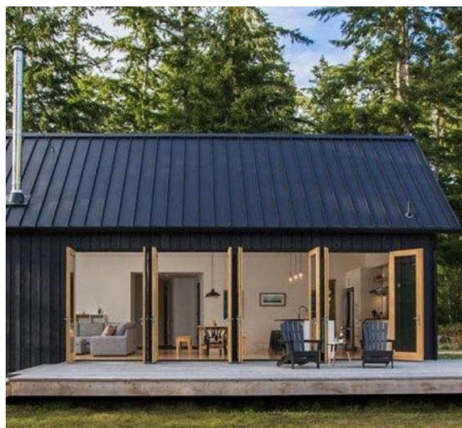
Fig08: Example of black timber cladding and black metal profiled roof
