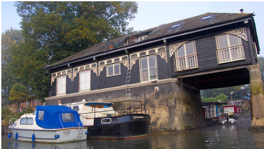
Fig06: Example of black timber cladding on Eel Pie Island
