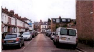
Current View with Gregg 3 storey building.
