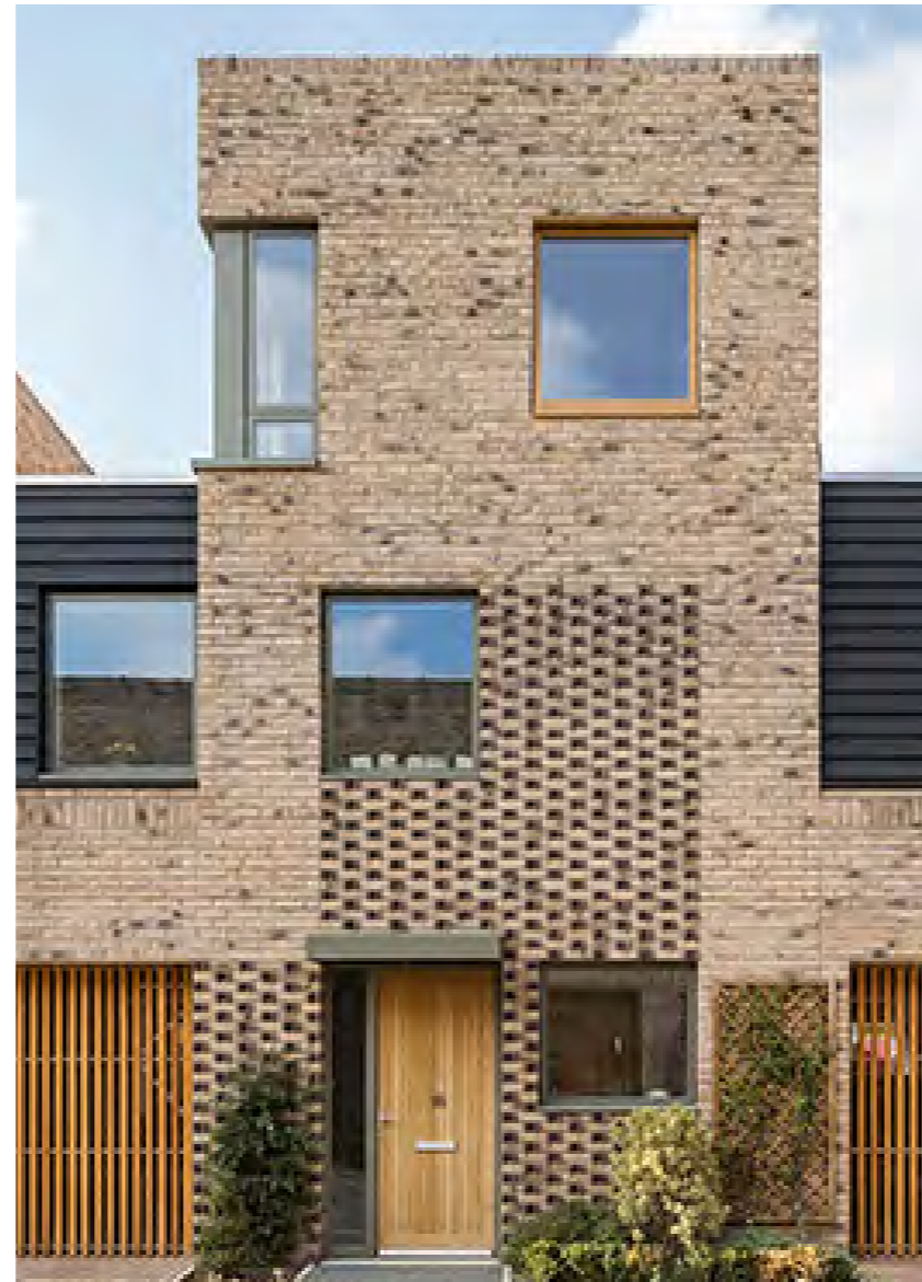
Example of timbers secondary elements only
