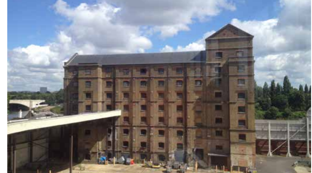
Photograph 5 - The southern facade of the Maltings.
