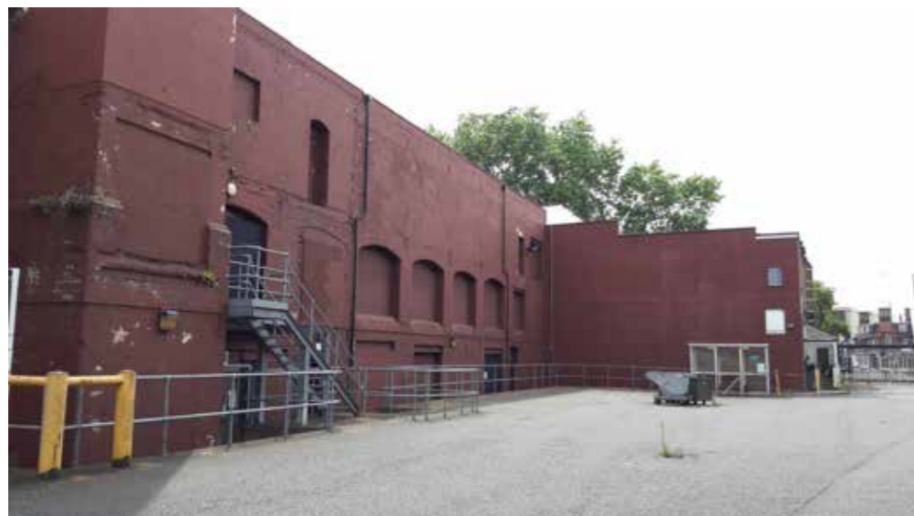
Photograph 6 - Former Hotel and Former Bottling Building.
