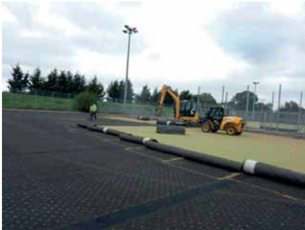
Rolling up carpet – limiting damage during process
