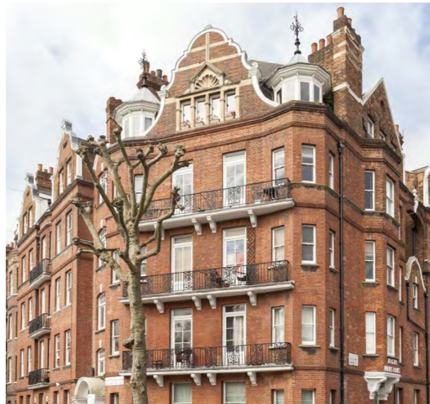
Digby Mansions (street facing facade)
