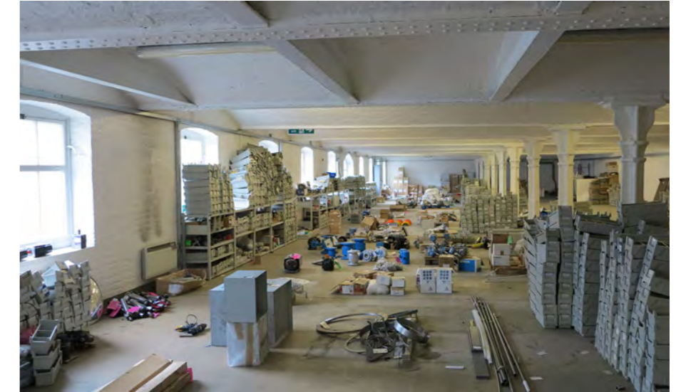
Existing photograph of vaulted structure to bottling building
