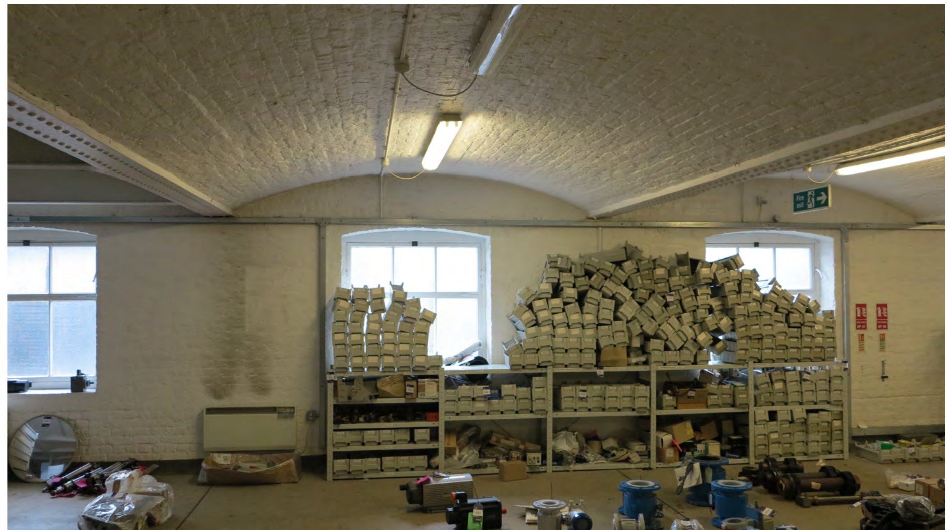
Existing photograph of vaulted structure to bottling building
