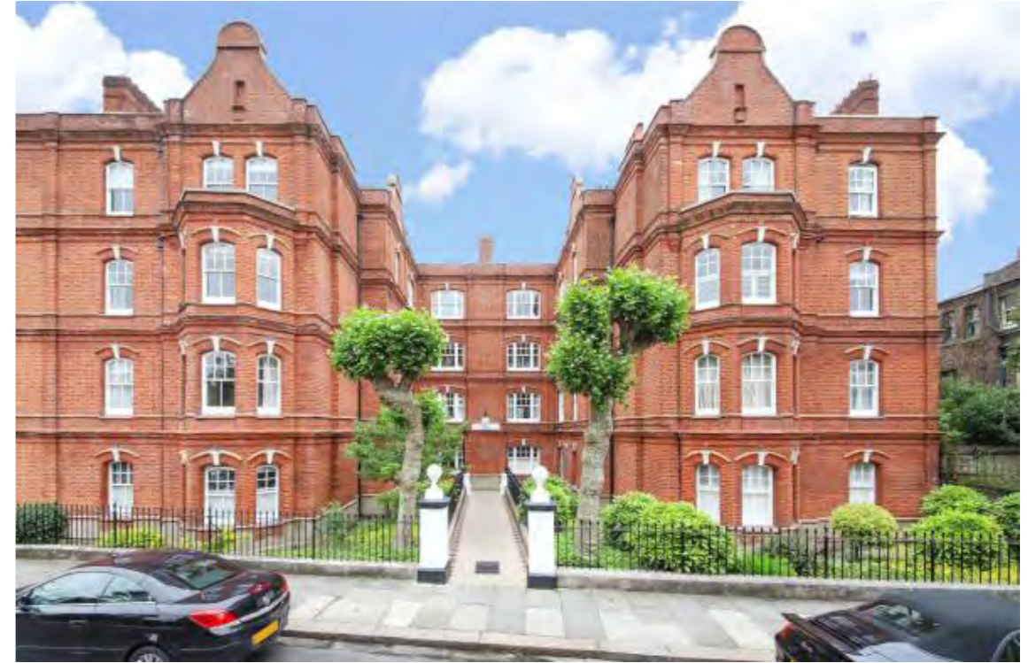
Exterior view of Queens Club Mansions
