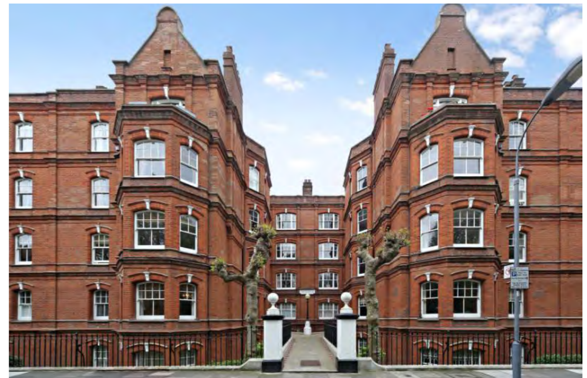
Exterior view of Queens Club Mansions
