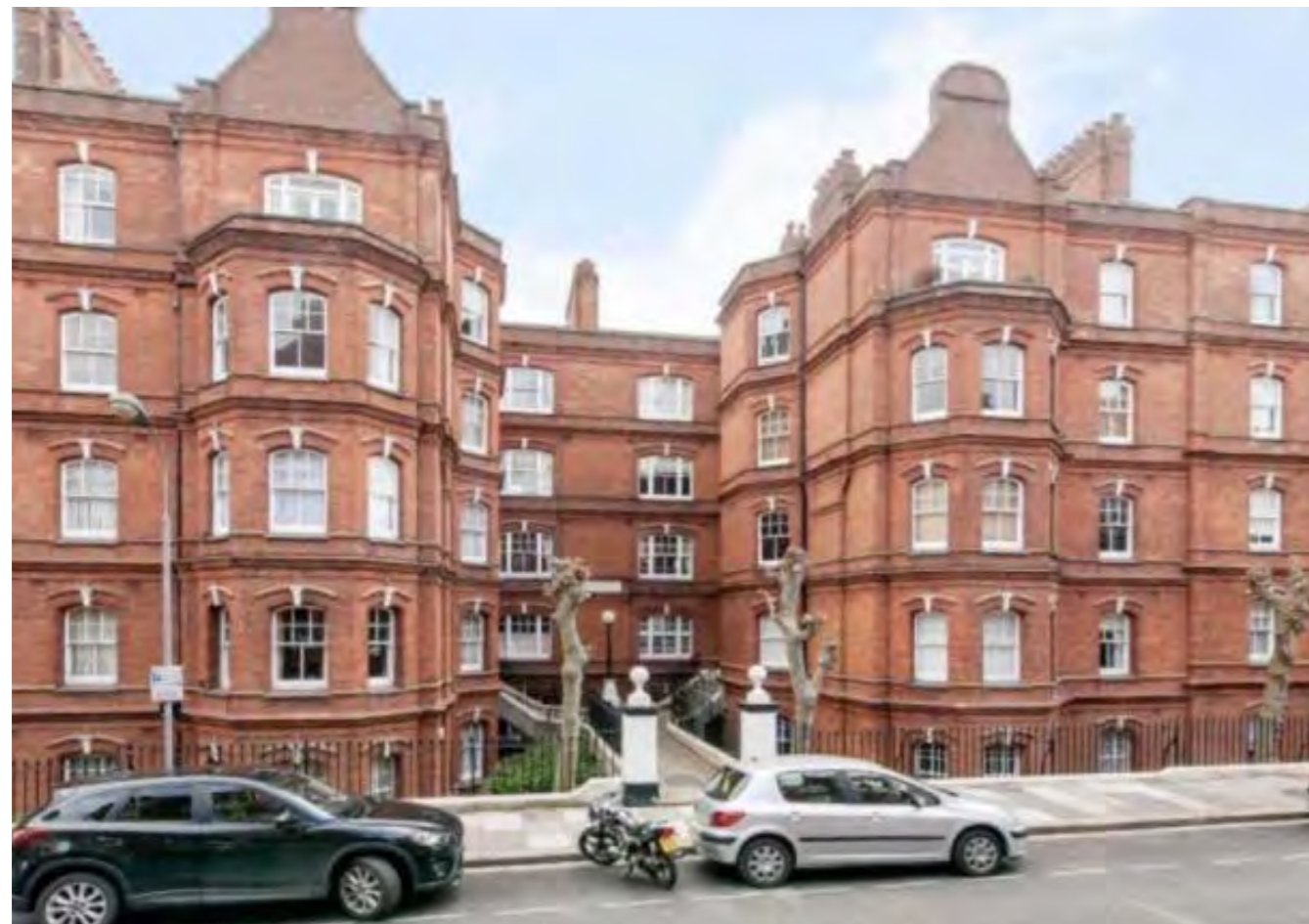
Exterior view of Queens Club Mansions
