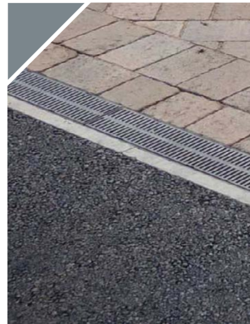
Hot Rolled Asphalt
