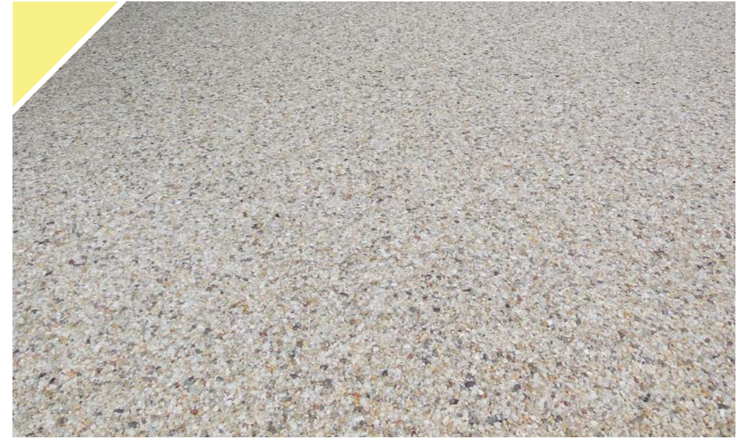
Resin Bound Aggregate Paving
