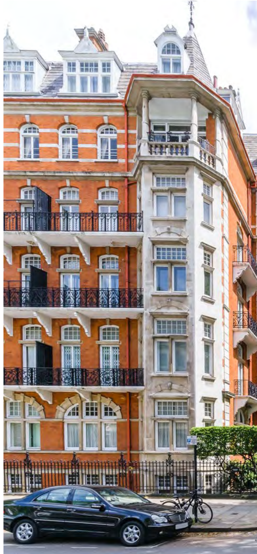
Alexandra Court - example of vertical hierarchy within balustrade design
