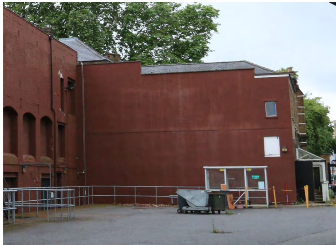
Existing east elevation of former hotel building
