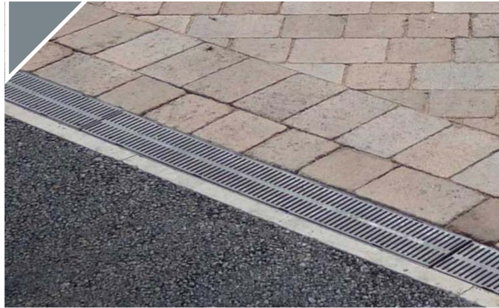
Hot Rolled Asphalt
