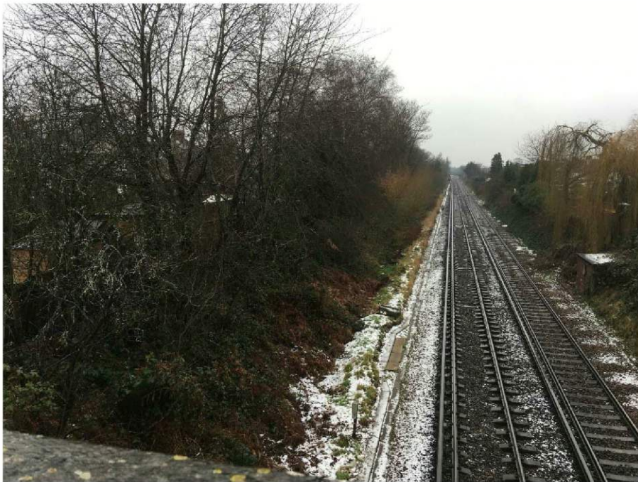
Photograph 2 – View west from Percy Road
