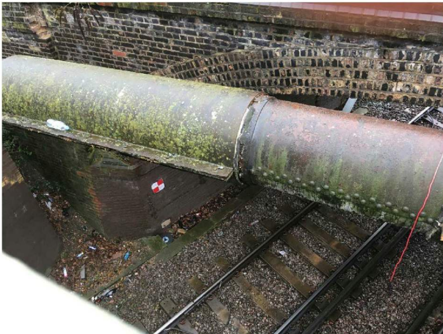
Photograph 4 – Railway beneath Hospital Bridge Road
