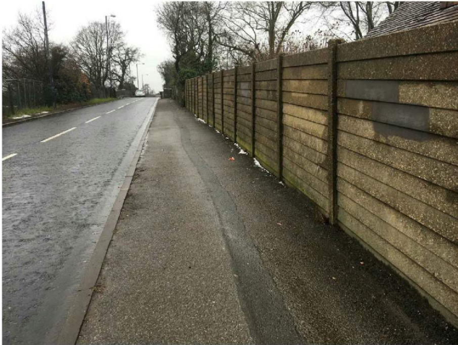
Photograph 3 – Hospital Bridge Road separating the waterbody from the Site
