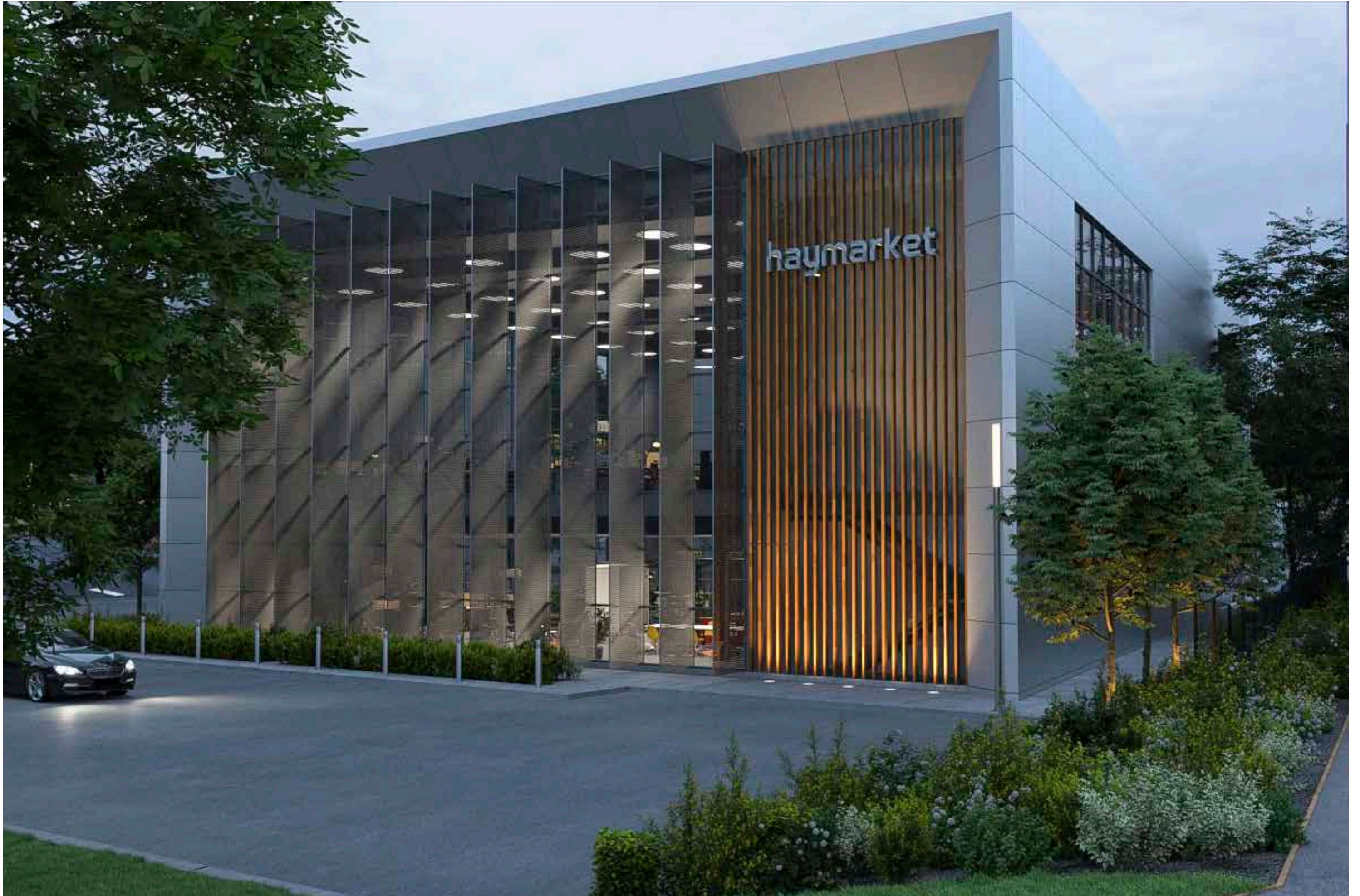
View of north elevation from Marsh Farm Lane
