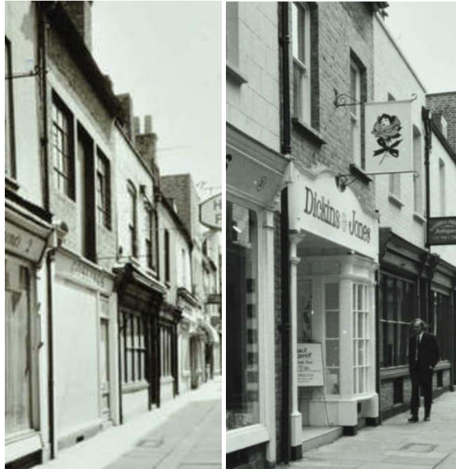
Figure 15: No. 4 Paved Court – (i) 1968, before shopfront and windows were replaced and (ii) 1972 after refurbishment
