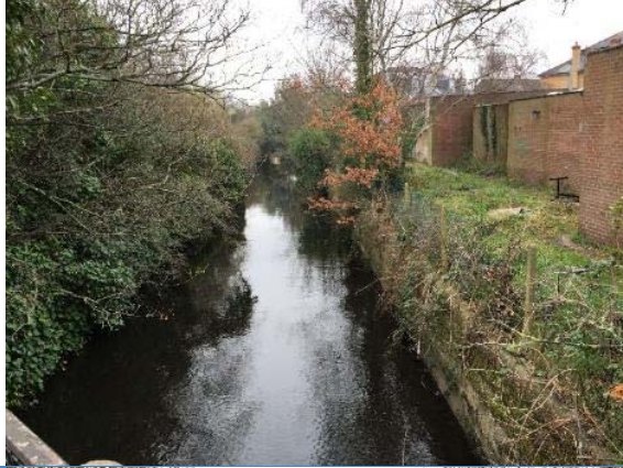
Photograph 8: section of River Crane showing scrub habitat and concrete lined banks (TN8)
