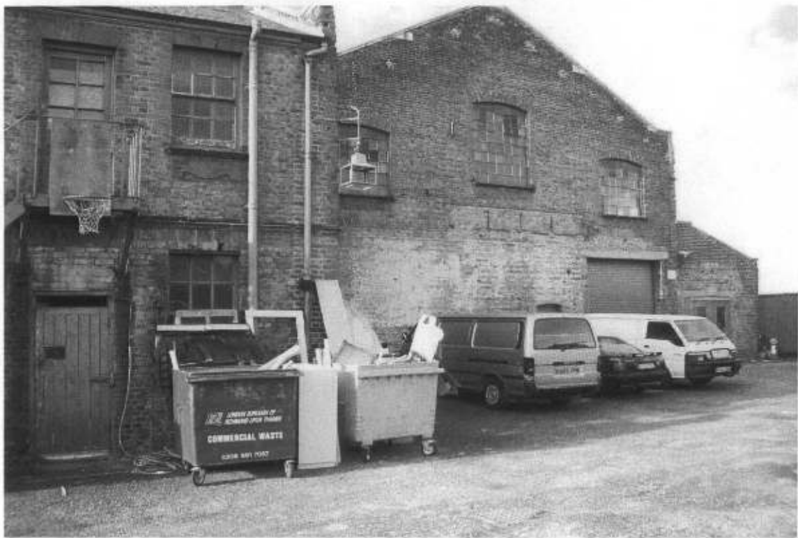
Fig. 11: The east elevation of the boiler house of the generating station at Hamilton Road, Twickenham
