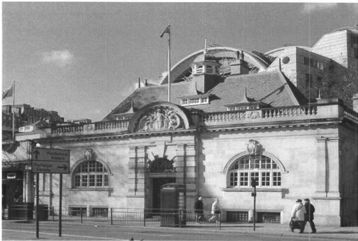
Fig. 7: London County Council generating station, Victoria Embankment
