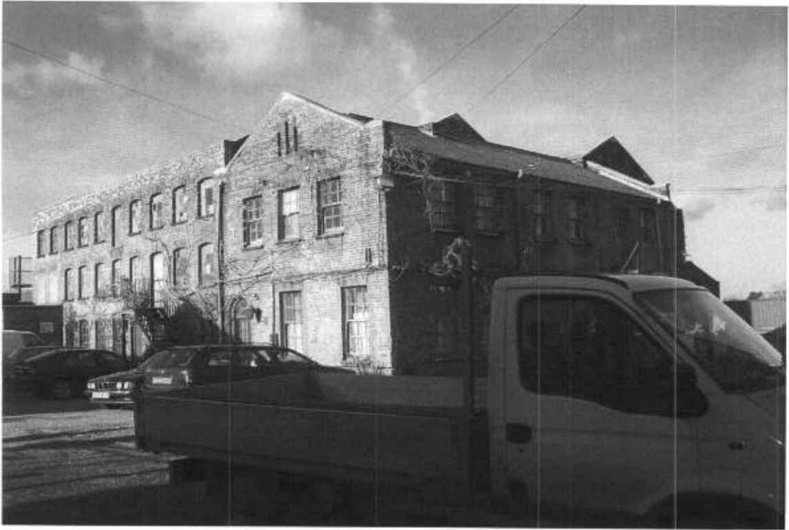
Fig. 9: The generating station at Hamilton Road, Twickenham, from the south-east
