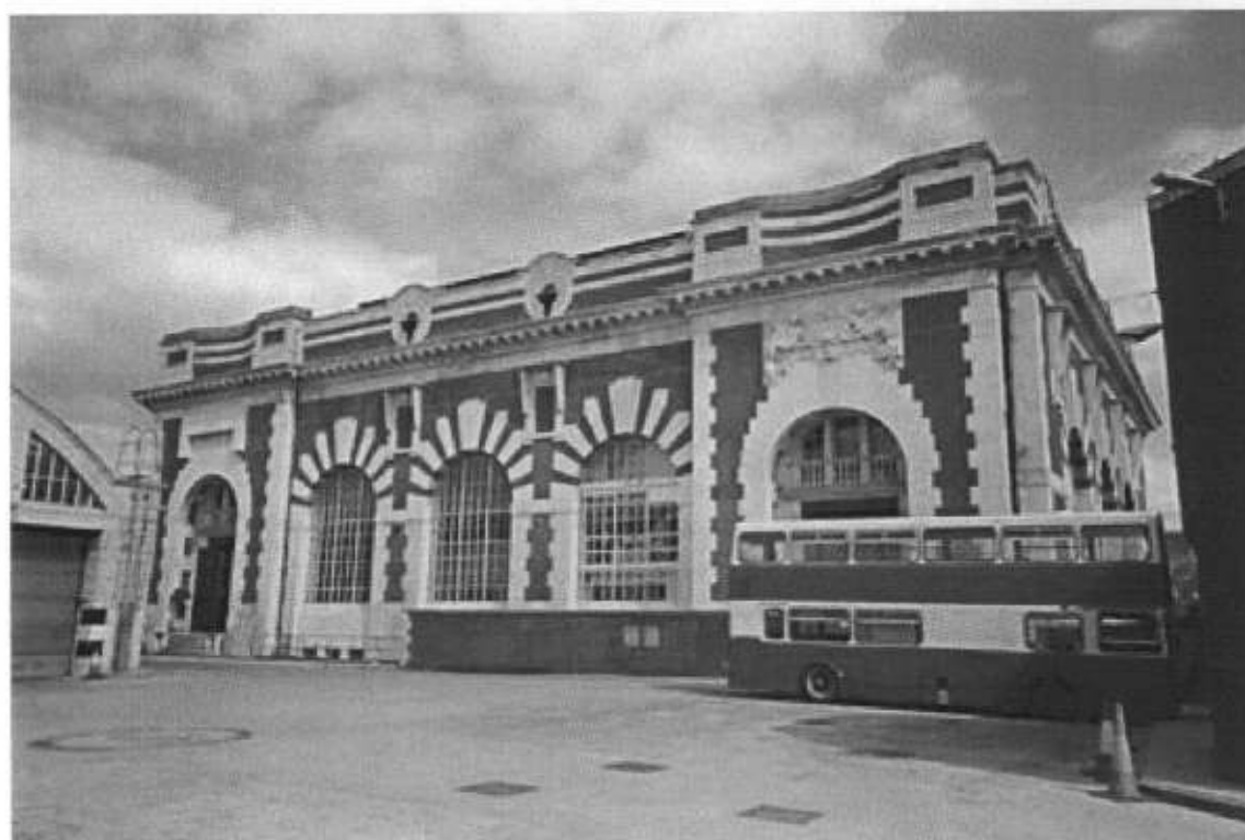
Fig. 5: London United Tramway Company generating station, Chiswick
