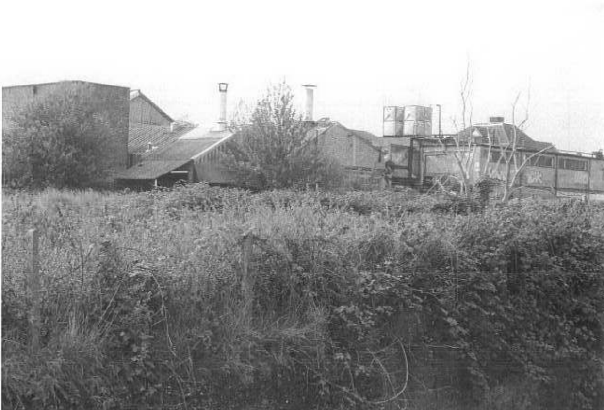
VIEW OF LARGER SCALE INDUSTRIAL BUILDINGS
