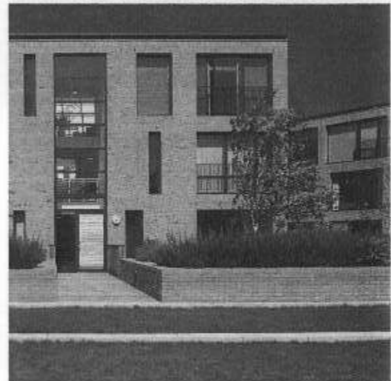
BENNET'S COURTYARD - MERTON - FEILDEN CLEGG BRADLEY
