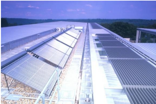
Evacuated tube solar thermal collectors (left) and average annual solar radiation (kWh/m 2 ) in the UK (right)
