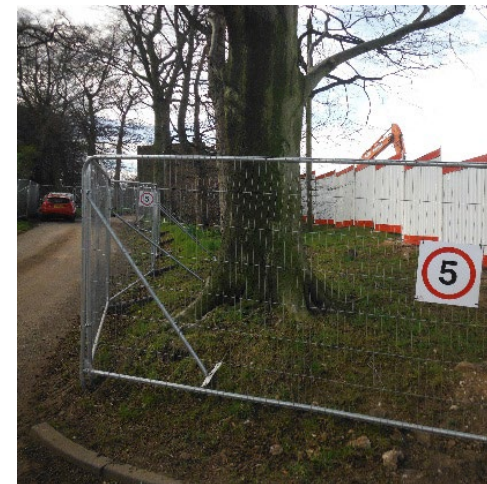
b) Stabilizer strut mounted on block tray
