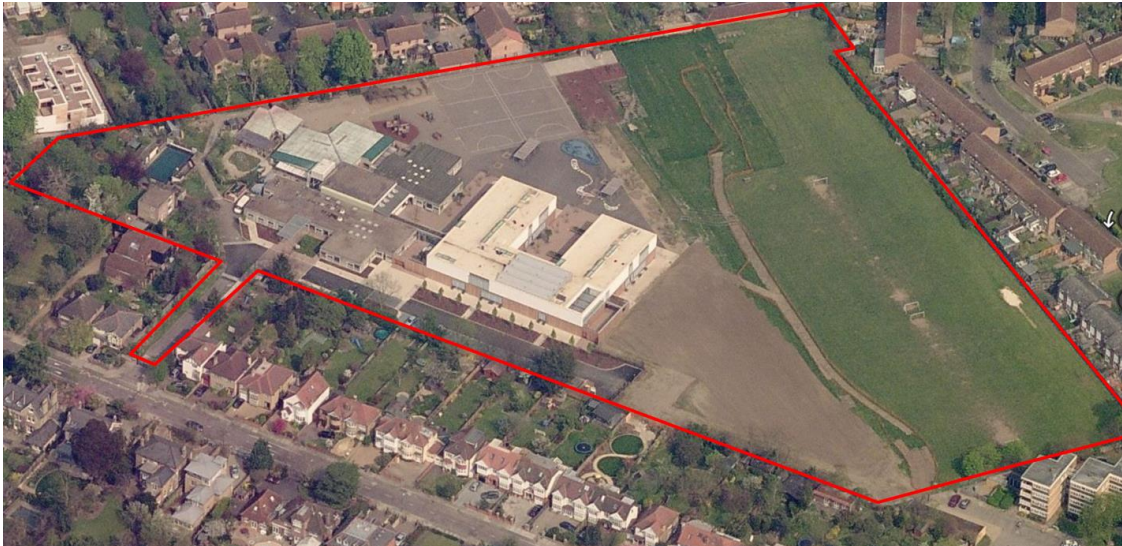
AERIAL VIEW OF COLLIS PRIMARY SCHOOL
