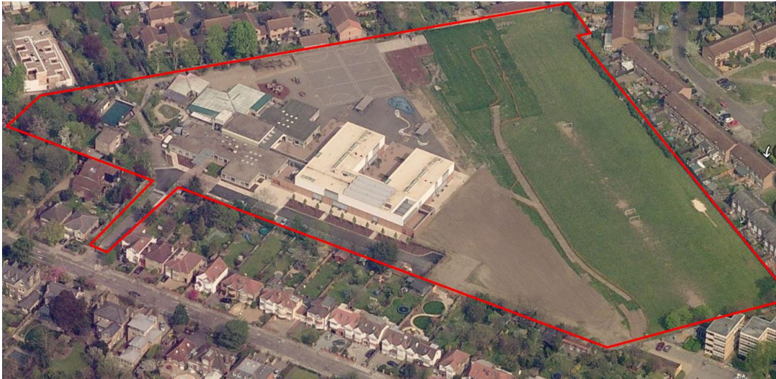
AERIAL VIEW OF COLLIS PRIMARY SCHOOL
