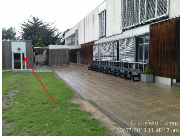
Figure 11: Rear elevation of B4.
