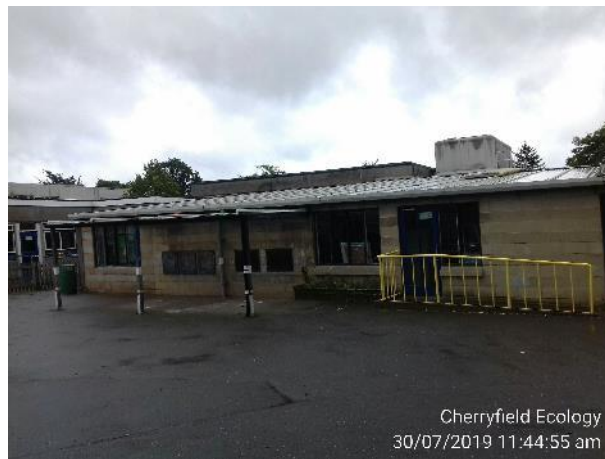
Figure 3: Rear elevation of B1.
