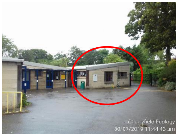
Figure 6: Rear elevation of B2.
