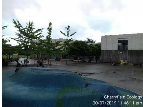
Figure 8: Rear elevation of B3.
