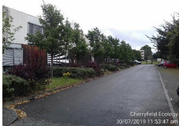
Figure 10: Front elevation of B3.
