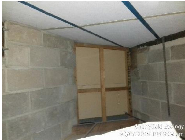
Figure 5: Example of B1 loft space.
