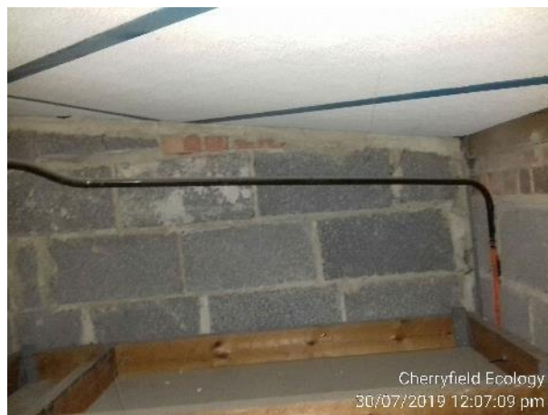
Figure 7: Example of B2 loft space.
