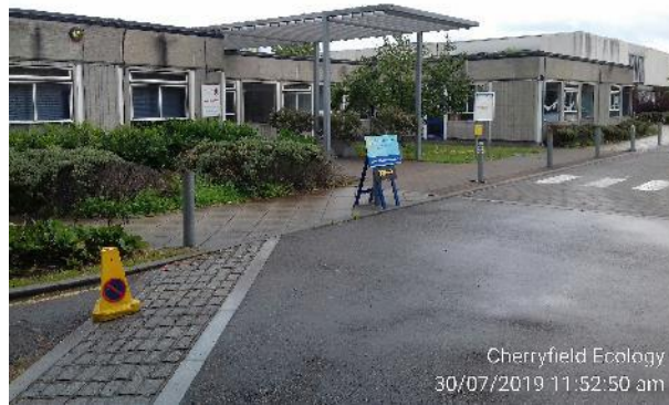
Figure 2: Front elevation of B1.
