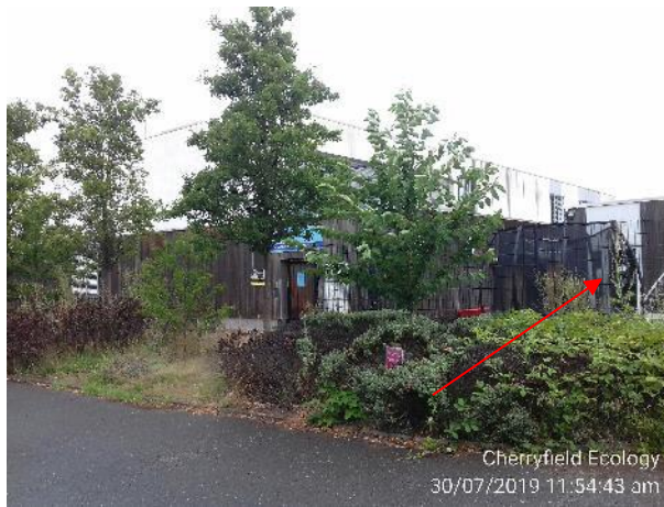
Figure 12: Front elevation of B4.
