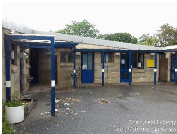
Figure 4: Rear elevation of B1.
