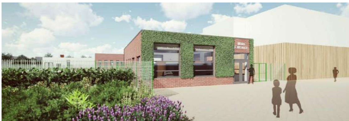
VISIBLE GREEN WALL FOR ADMIN/ENTRANCE BLOCK
