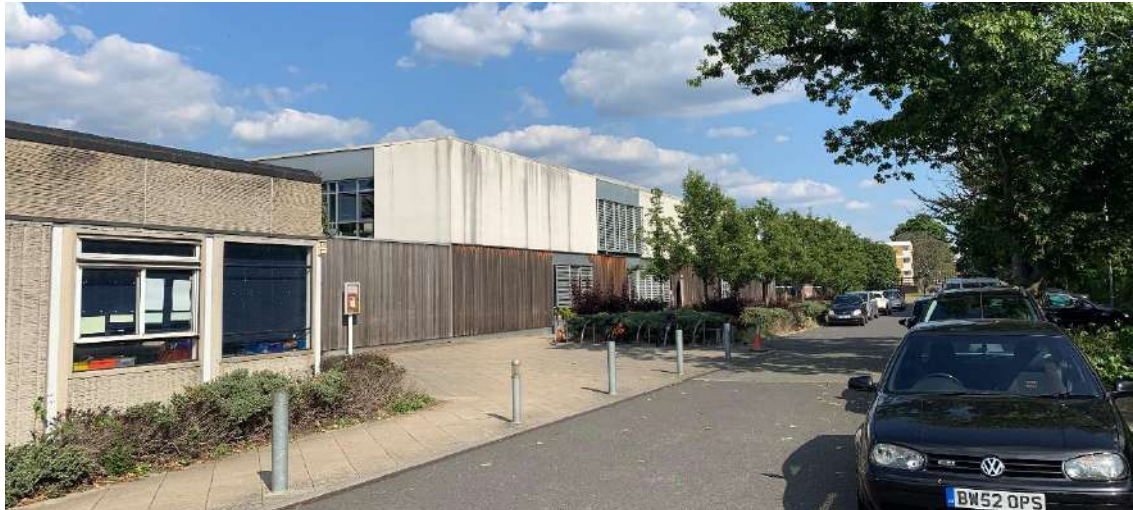
2 STOREY BLOCK EFA-B VIEWED FROM THE CAR PARK
