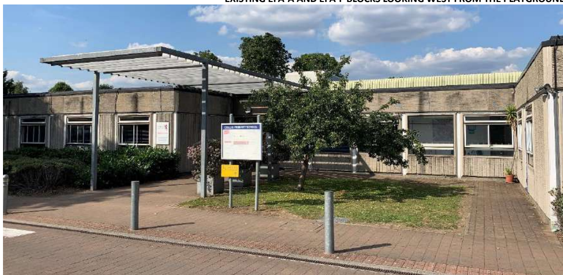
ENTRANCE TO BLOCK EFA-A WHEN VIEWED FROM THE CAR PARK
