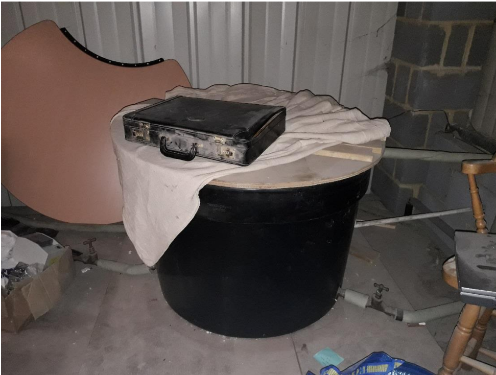
Photo 3: A <500 litre capacity water butt stored on the mezzanine level within the commercial area.
