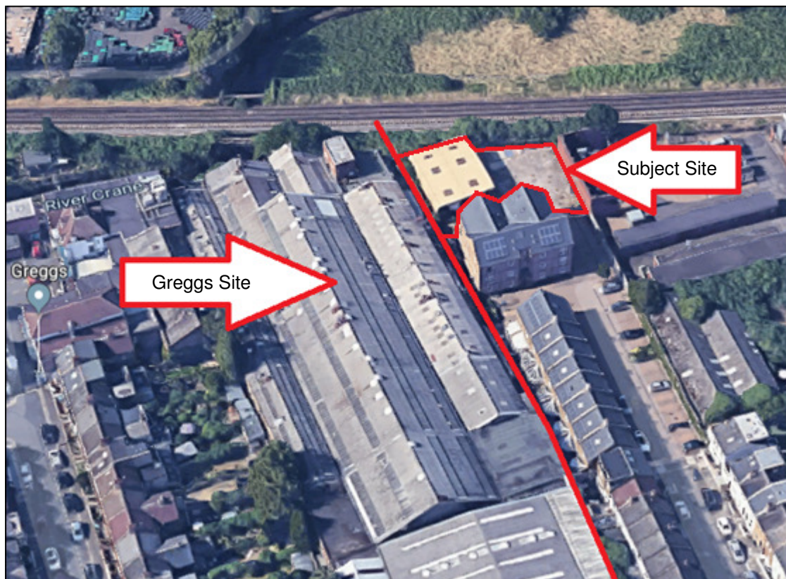
Aerial view demonstrating the relationship between the subject site and the Greggs site.
