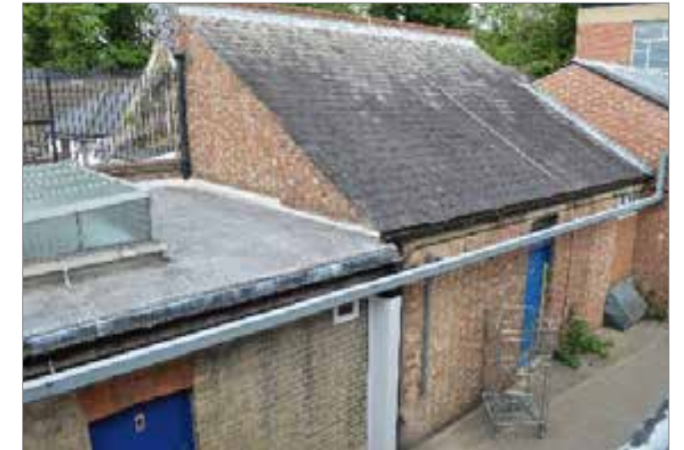
The existing link block (left and shed to western rear wing)
