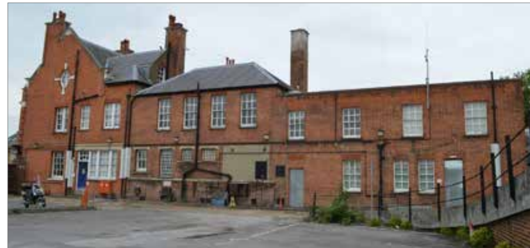
The east facade of the existing building
