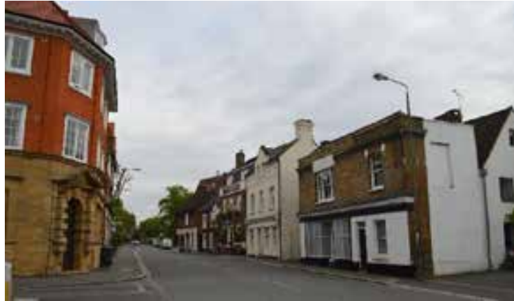
View of properties along the High Street
