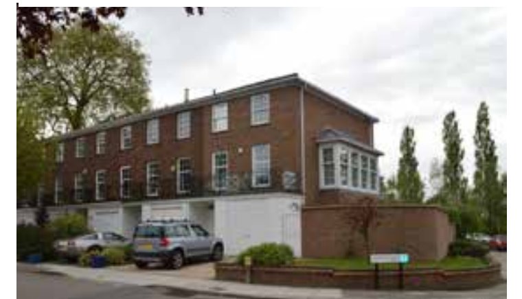
Johnson's Drive off the High Street
