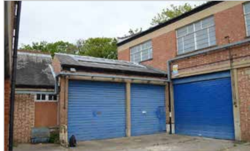
The sheds and garages to the north west corner of the site
