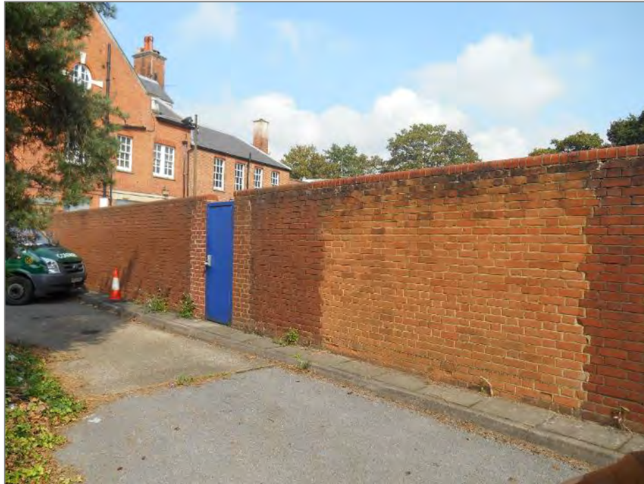
Photo 11: Front of Police Station
