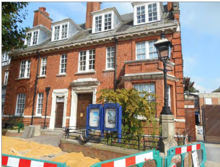
Photo 10: View of Police Station from Station road
