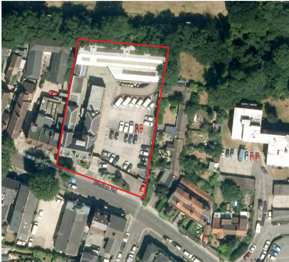
Figure 2: Aerial photograph of the site showing the approximate site boundary
