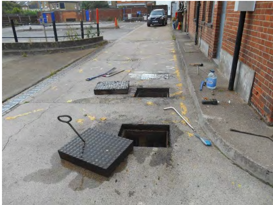
Photo 37: Underground drainage pipes
