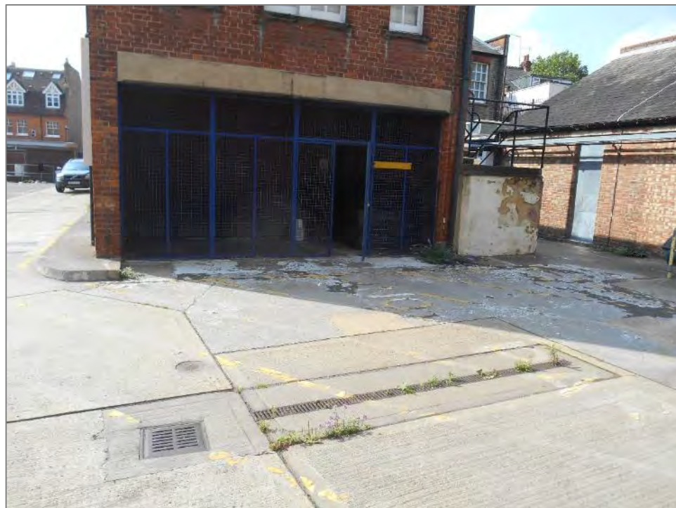
Photo 22: Location of the two smaller underground fuel storage tanks located at the rear of the station
