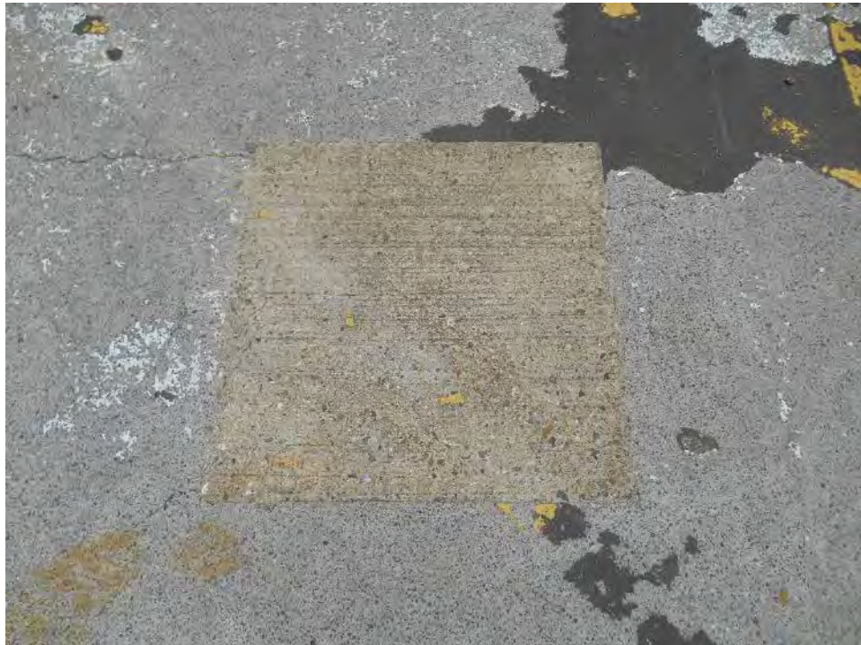
Photo 35: Underground fuel storage tank located at the rear of the station
