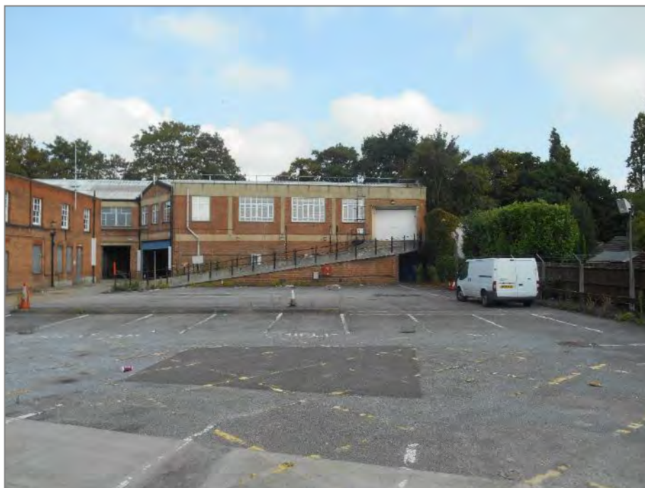
Photo 2: Police Station car park
