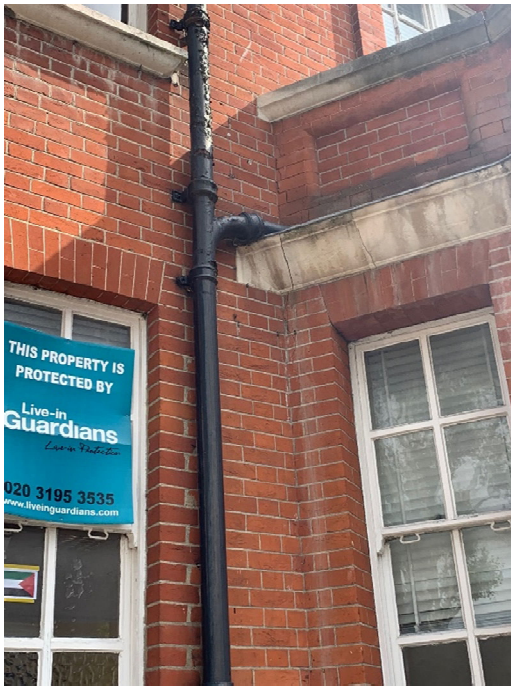
6. Junction of main walls to bay window – front elevation
