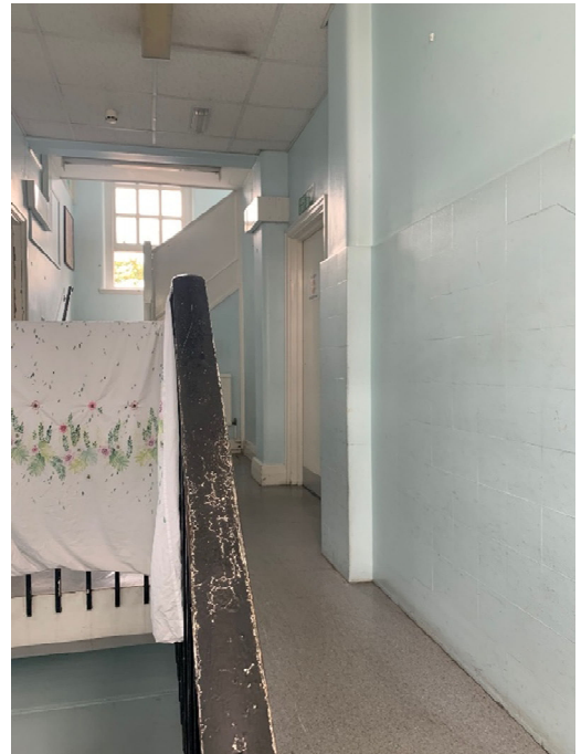
9. Column casements adjacent staircore at first floor
