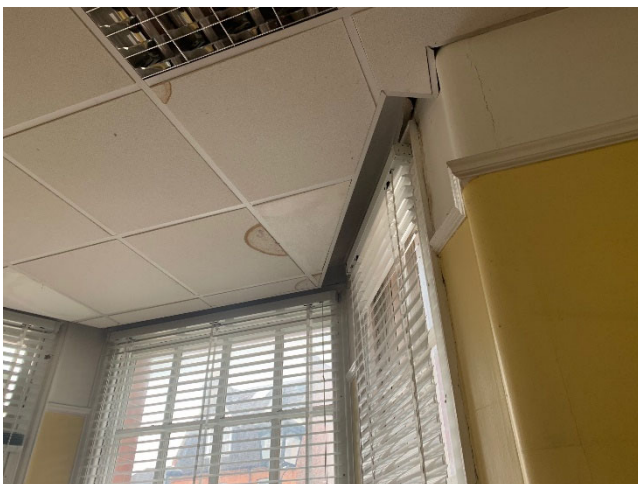
8. Internal view of ground floor bay window
