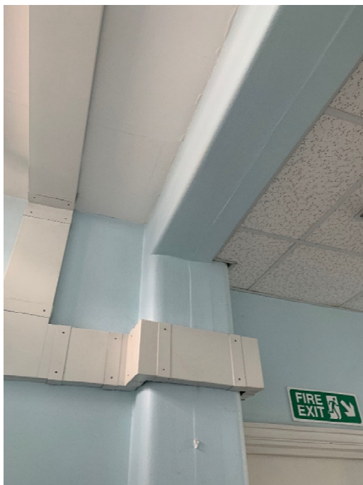
12. Column casement and downstand beam adjacent staircore at first floor
