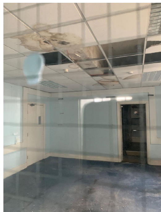
7. Downstand beam adjacent single storey rear extension
