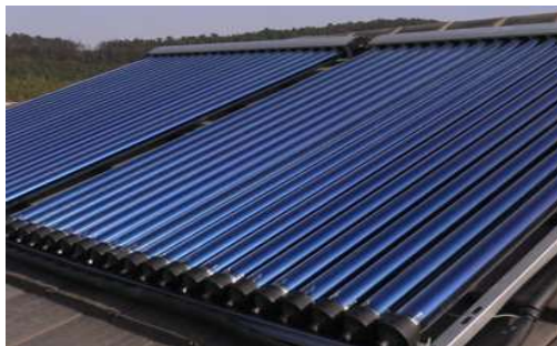
Figure 5 - Evacuated tube solar thermal panels
