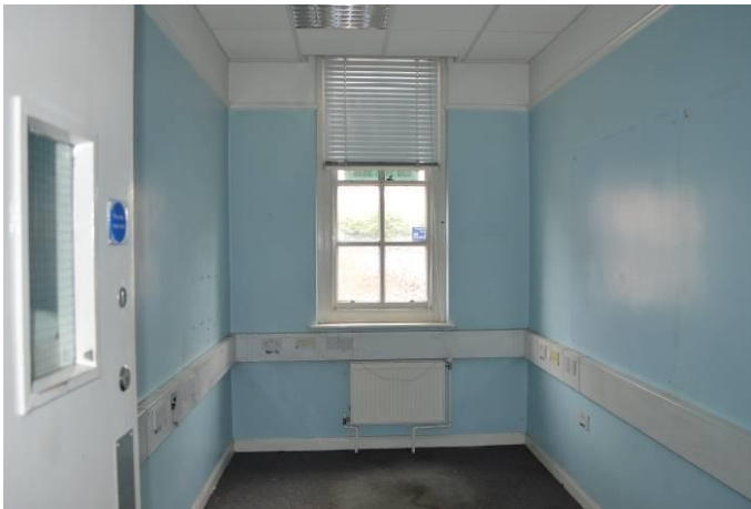
A typical room with modern suspended ceiling, fire door, service trunking, etc.
