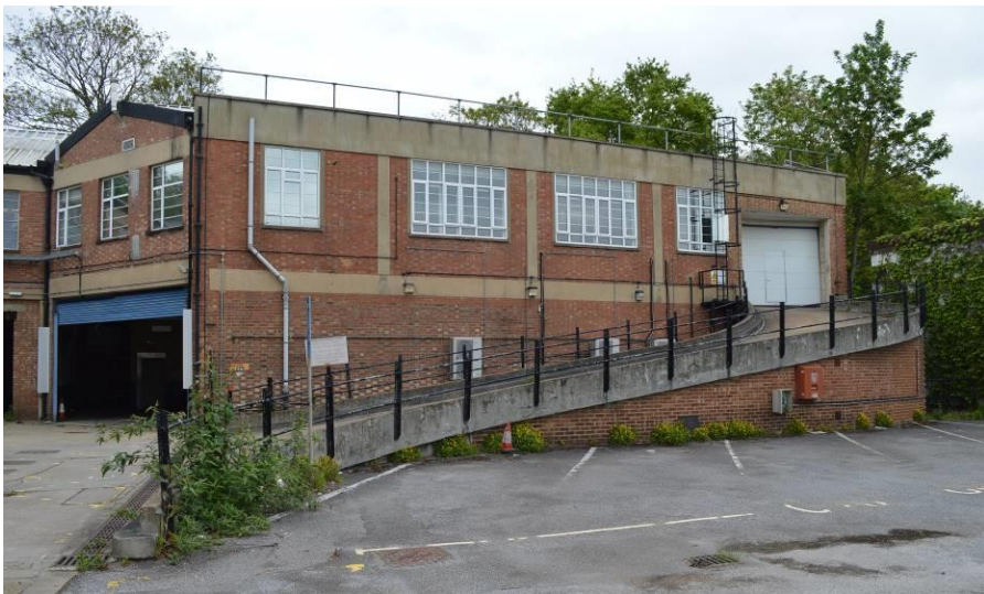
The 1930s garage and postwar ramp at the rear of the site.
