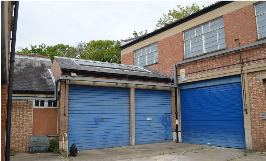
The 1930s sheds and garages in the north west corner of the site.
