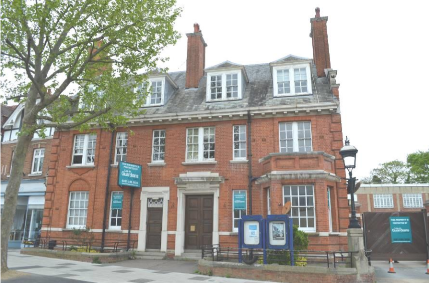
The front façade of the 1905 building.
