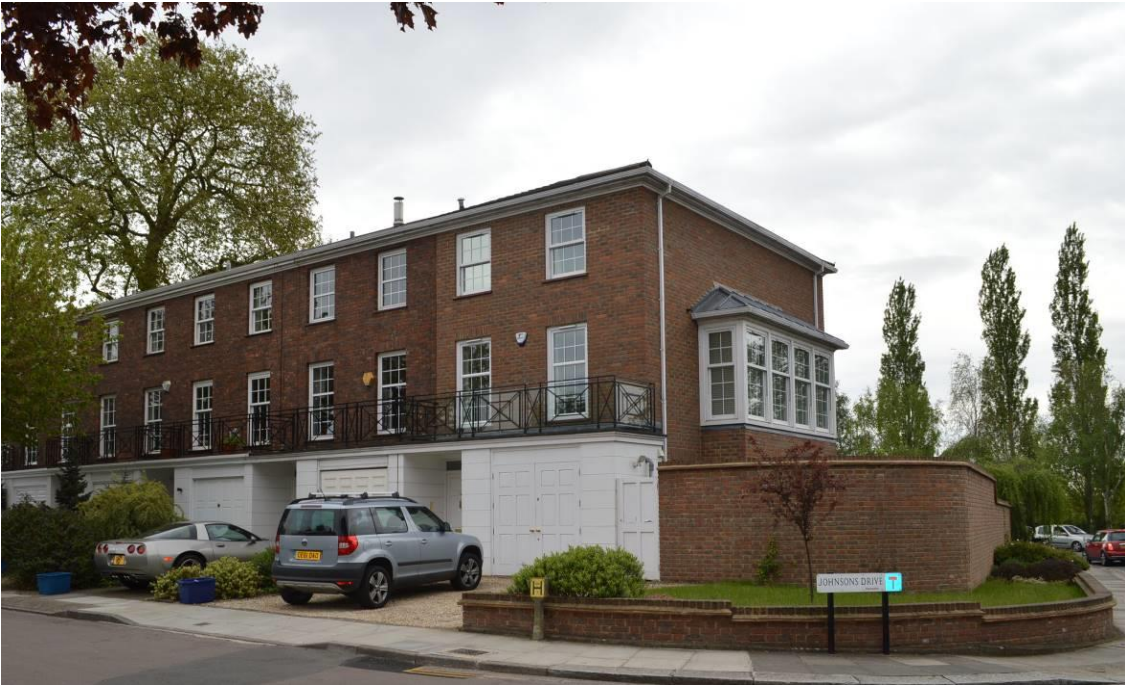
Modern housing with traditional features on Johnson’s Drive, off the High Street.
