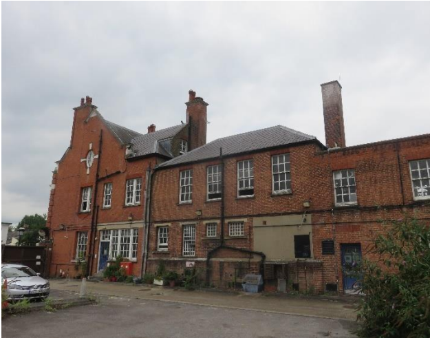
Plate 9.1: Buildings present on site
