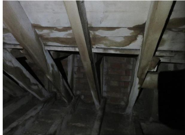
Plate 4.12: Boarding Concealing Brickwork
