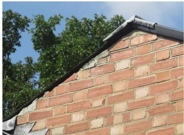
Plate 4.14: Missing Mortar at Gable End
