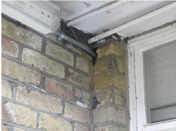
**Plate 4.7: Holes in Brickwork**
