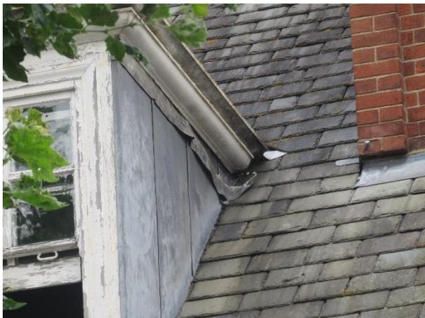
Plate 4.3: Lifted Lead Flashing
