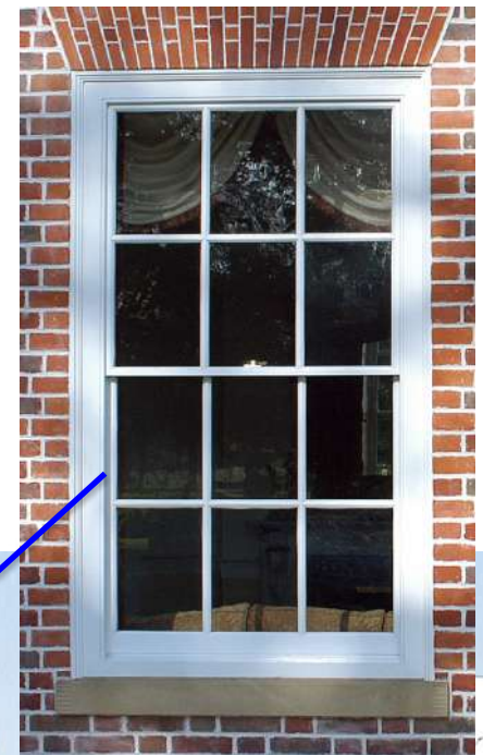
TIMBER DOUBLE GLAZED SASH WINDOWS
