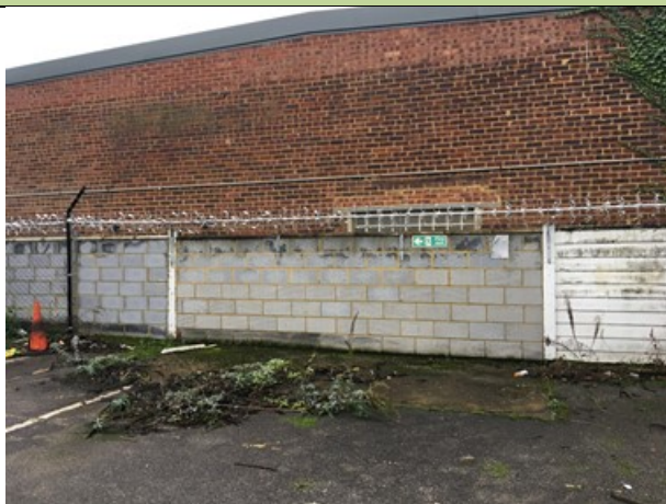
Photo 9: Examples of walls
