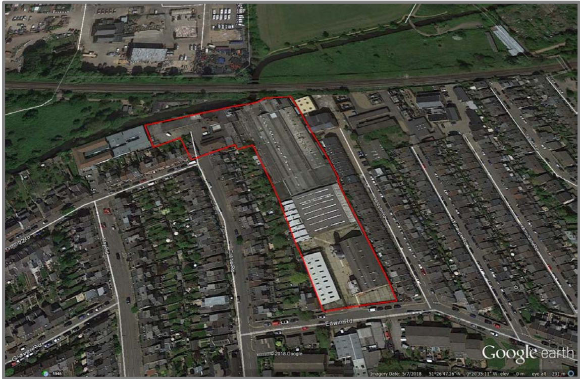
Figure 2: Aerial Mapping indicating the Greggs Bakery Site (outlined in red) © Google Earth 2019
