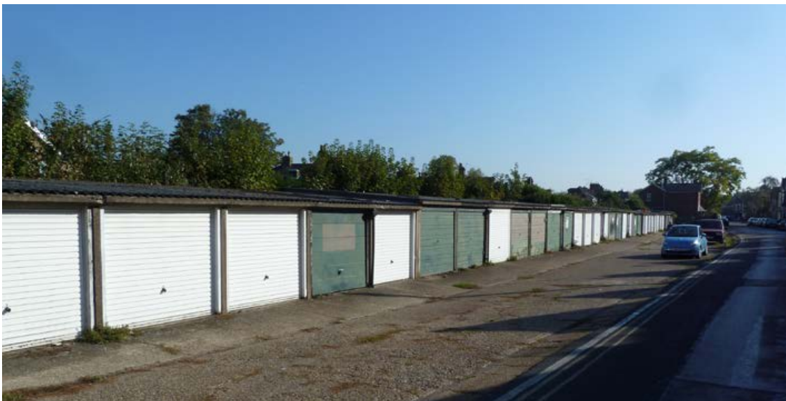
View of application site
