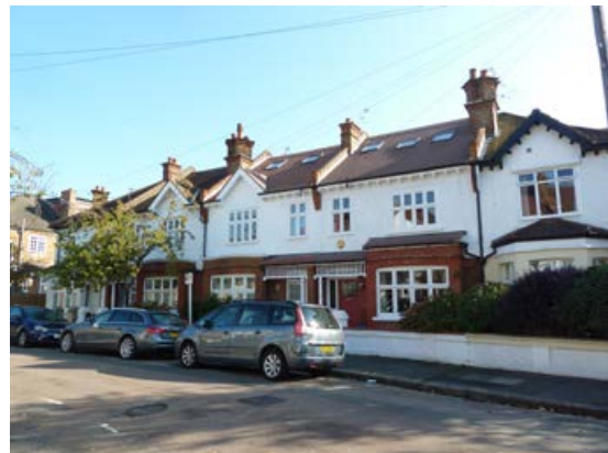
Terraced dwellings on Clendover Road
