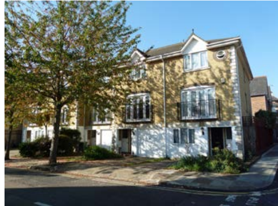
Terraced dwellings on Howgate Road
