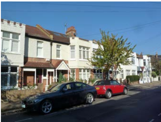
Terraced dwellings on Church Avenue
