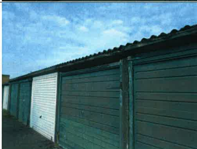
Photograph 5: A dislodged wood fascia board along the southern aspect of one of the garage units.
