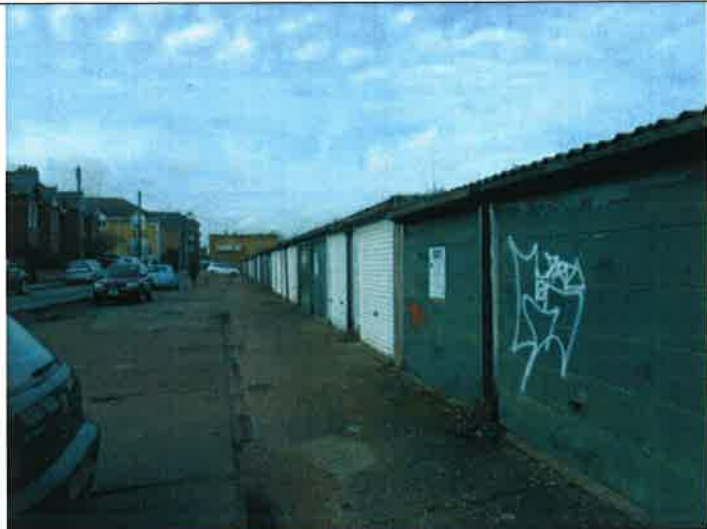
Photograph 1: An overview of the hard-standing and garage units on site.
