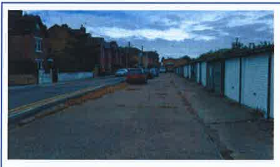
View west across front hardstanding area
