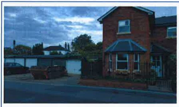
Eastern end of site and adjacent dwelling
