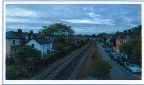
View from nearby footbridge – site on LHS in distance
