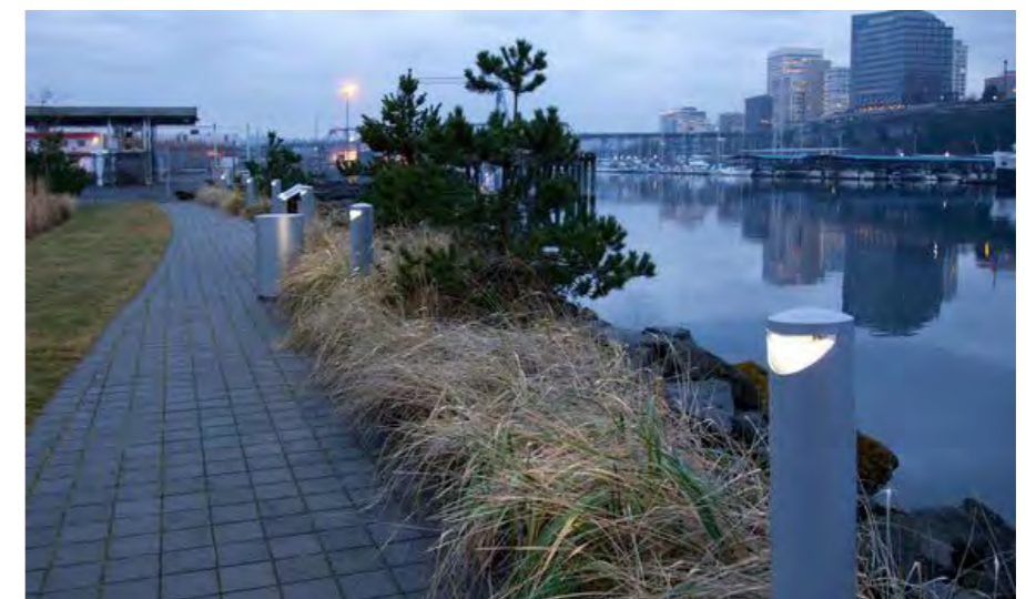
Example of bollard lighting
