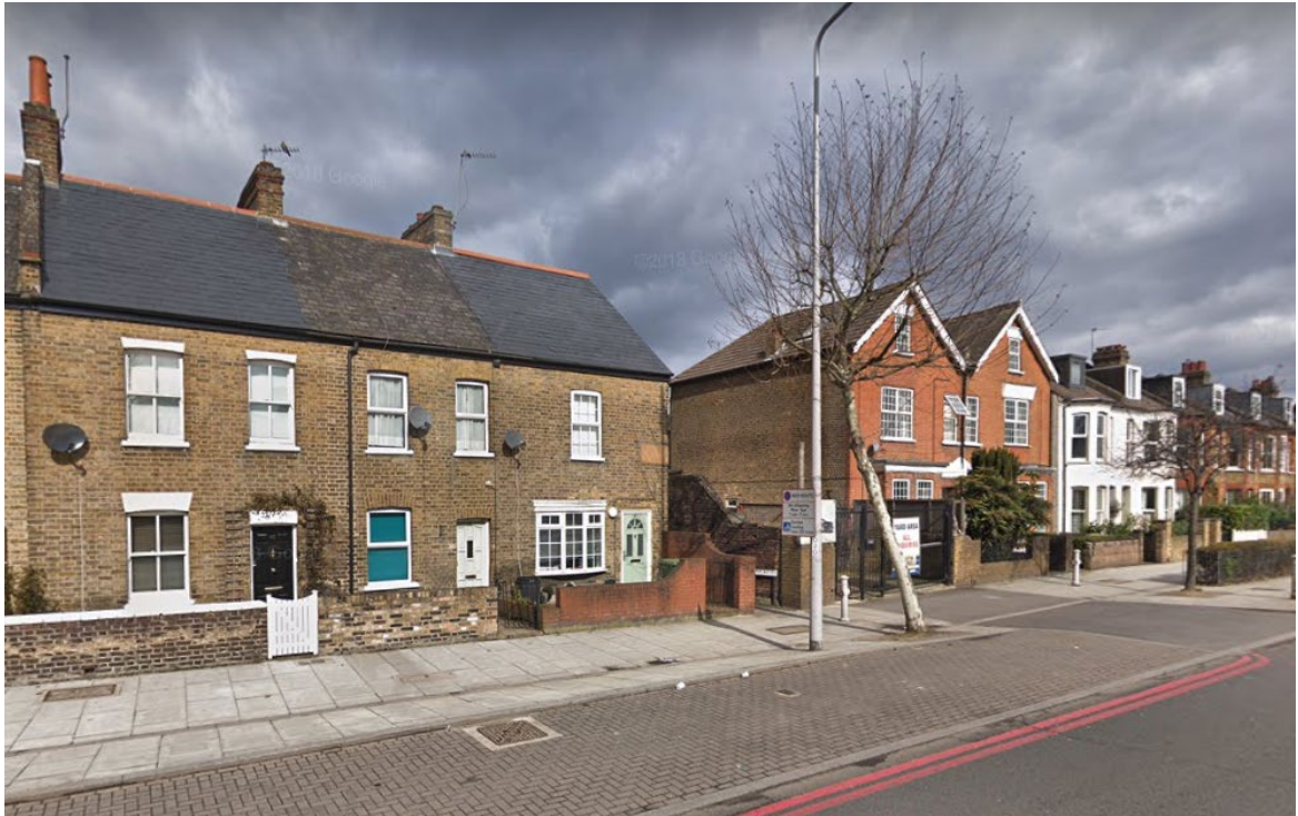
Figure 2. View of the Site from Lower Mortlake Road. From Google View March 2018 (no foliage).
