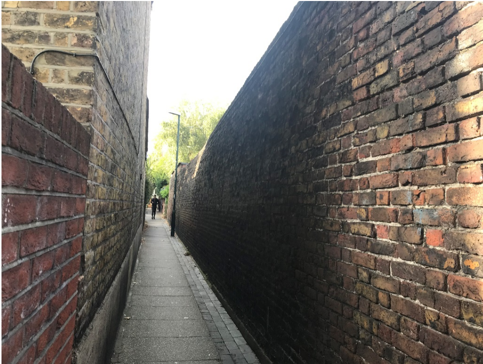
Appendix 3.5. Photograph showing the view along Blue Anchor Alley (the Site is located on the right)
