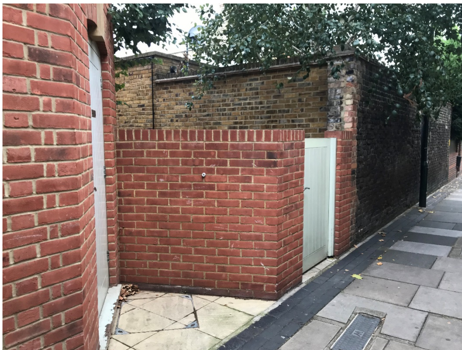
Appendix 3.4. Photograph showing the recent development at the northern extreme of Blue Anchor Alley (which provides precedent for the proposals)
