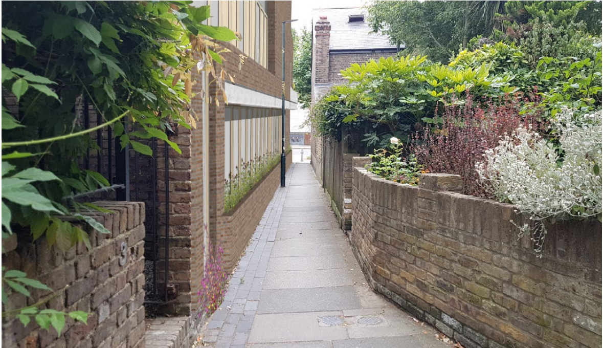
Figure 6. Visualisation of the proposed scheme along Blue Anchor Alley, looking south (the proposed building is on the left) ©Lynas Smith Architects
