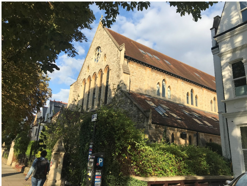
Appendix 3.12. Photograph showing Christ Church on Kew Road, a landmark building
