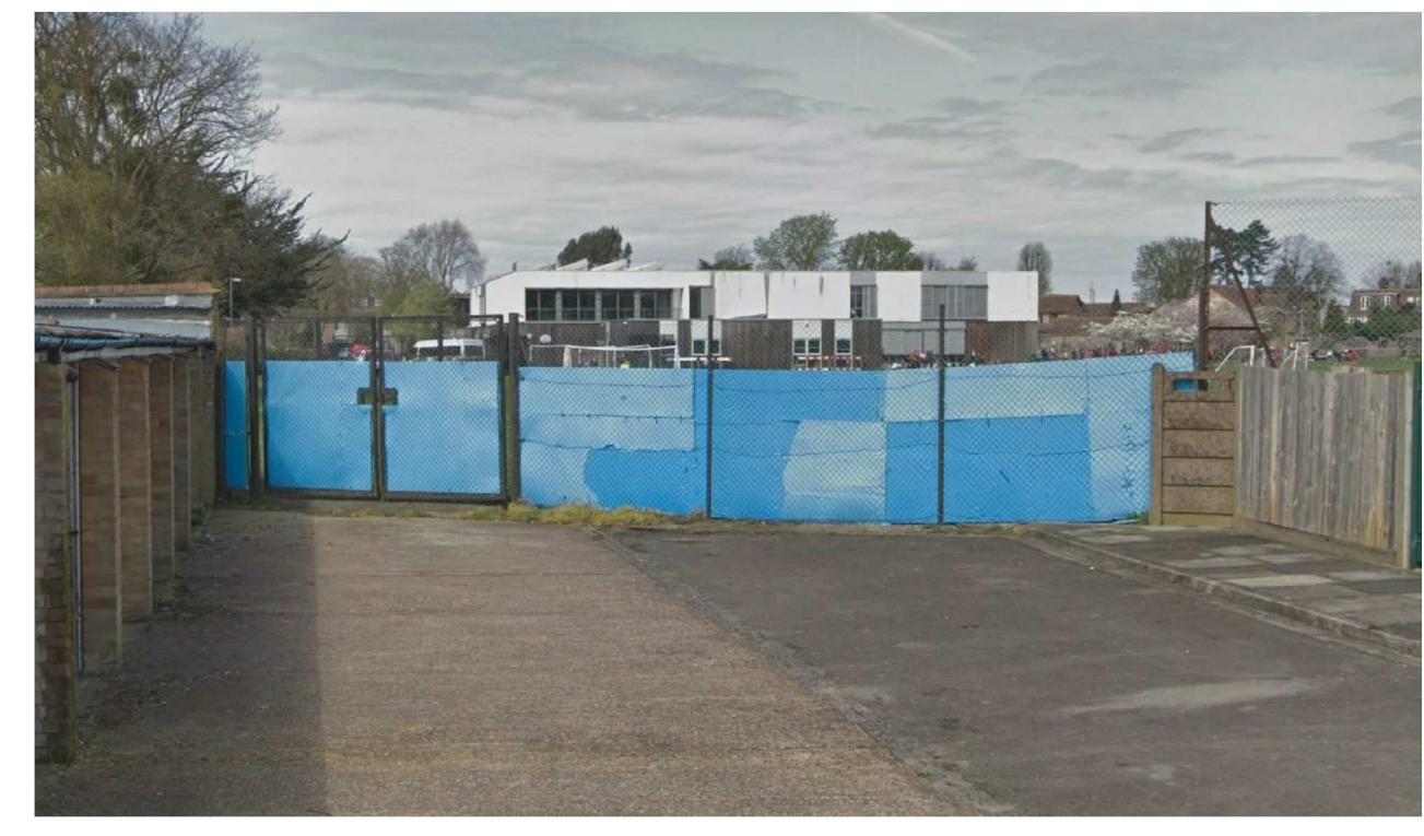
Image 03-SI Existing Site Gate Location Image taken from Google Maps 2019-10-23
